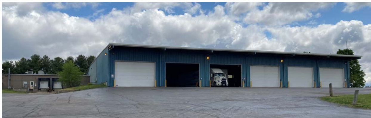
Figure S-14 CSB-2 (foreground) and CSB-1 (rear left) at the Clean Harbors Pocatonia Site
