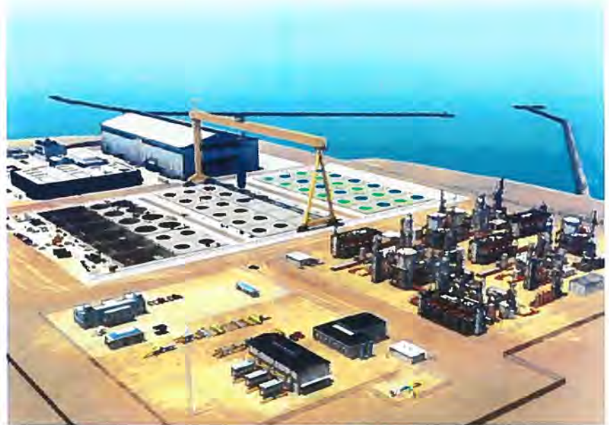
Fig. 2. Hydrogen gigafactory with factory in back, reactor field in the middle, and hydrogen plant in the front. (Image: LucidCatalyst)
