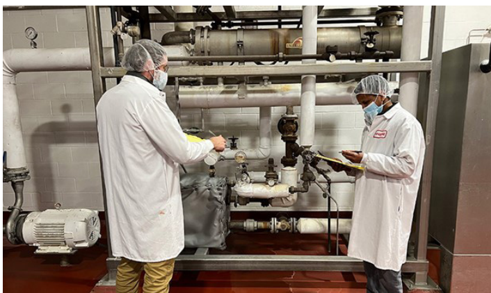
Assistant Director Ryan Swanson (left) and graduate student Tsegahaimanot “Andy” Andegiorgis (right) taking data at a steam-to-hot water heat exchanger during an audit. All photos courtesy of SFSU
