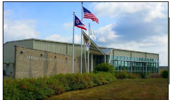
Fernald Preserve Visitors Center near Hamilton, Ohio.
