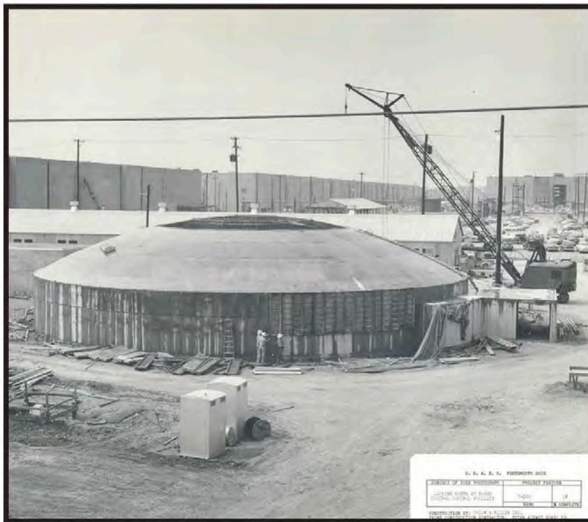
**Figure 14:** Construction Photo of the X-300 Plant Control Facility, May 1954
