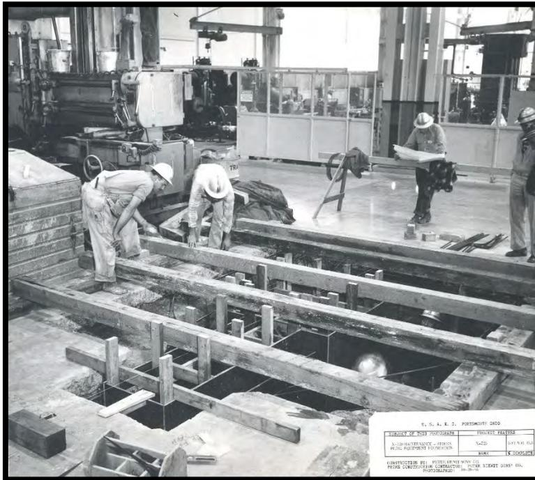
**Figure 22:** The X-720 Maintenance and Stores Building Equipment Foundation, October 1955
