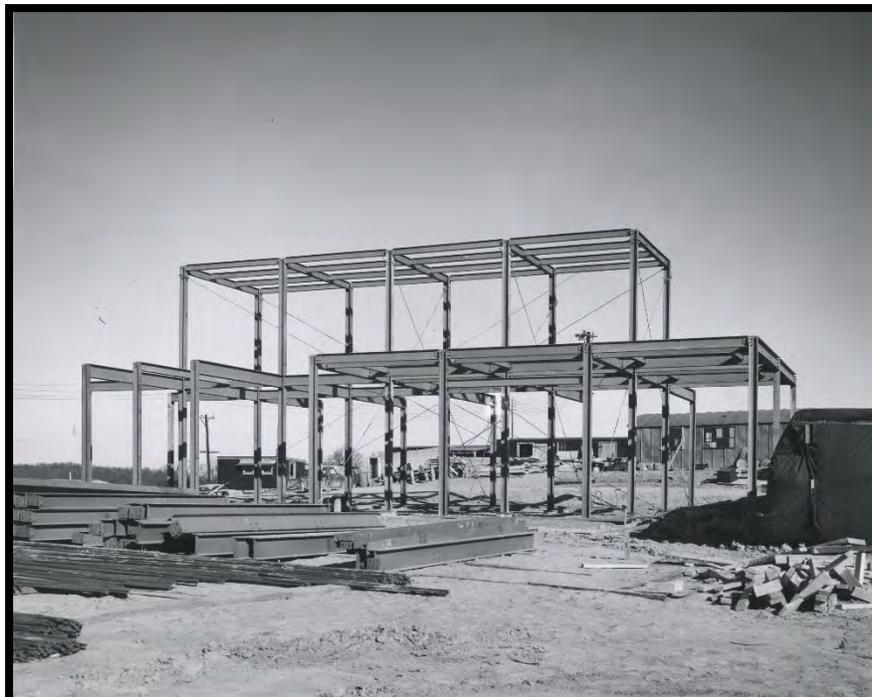
**Figure 9:** Steel Framework for the X-611 Water Treatment Plant
