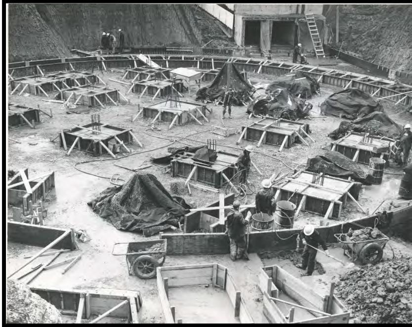
**Figure 5:** Construction Photo of the X-300 Plant Control Facility, January 1954
