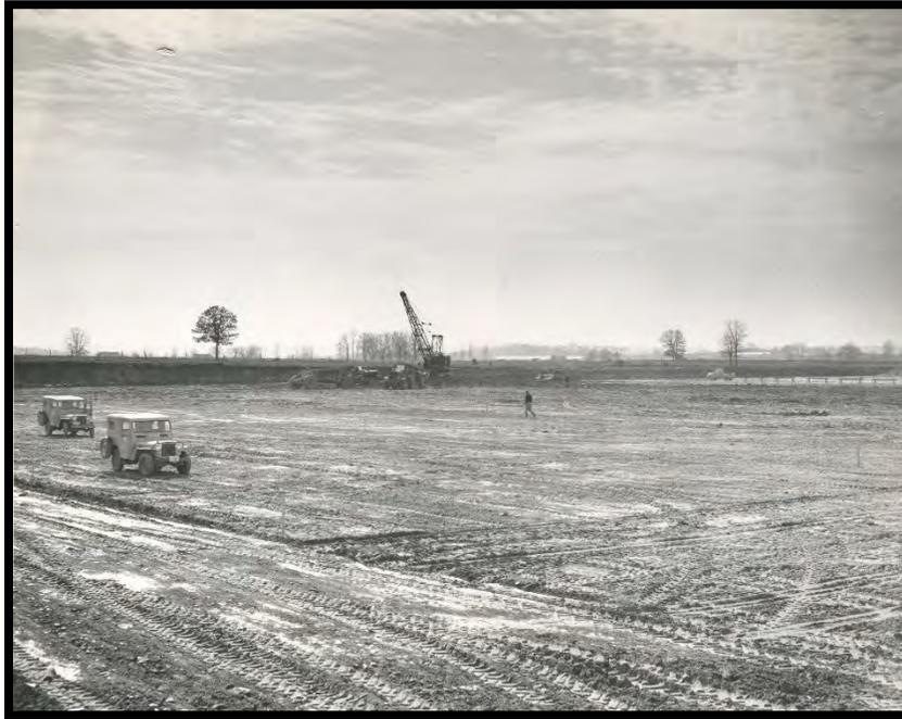
**Figure 4:** Grading Work for the X-720 Maintenance and Stores Building,
