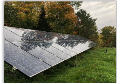
Figure 33: Men's Transitional Living Solar PV system
