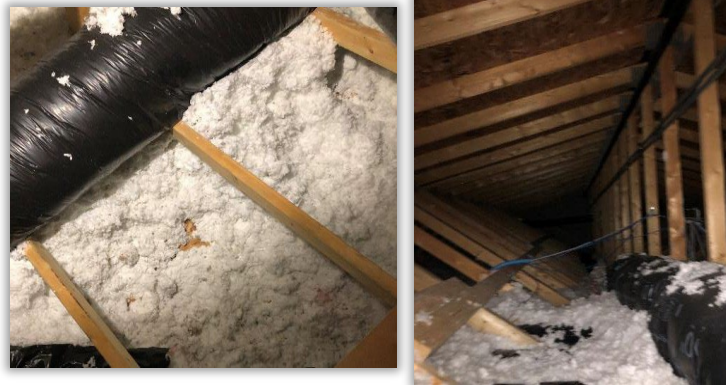
Figure 26: Caring Place Blown-In Insulation
