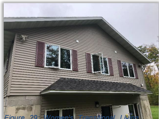
Figure 29. Women's Transitional Living Facility's Windows are Open
