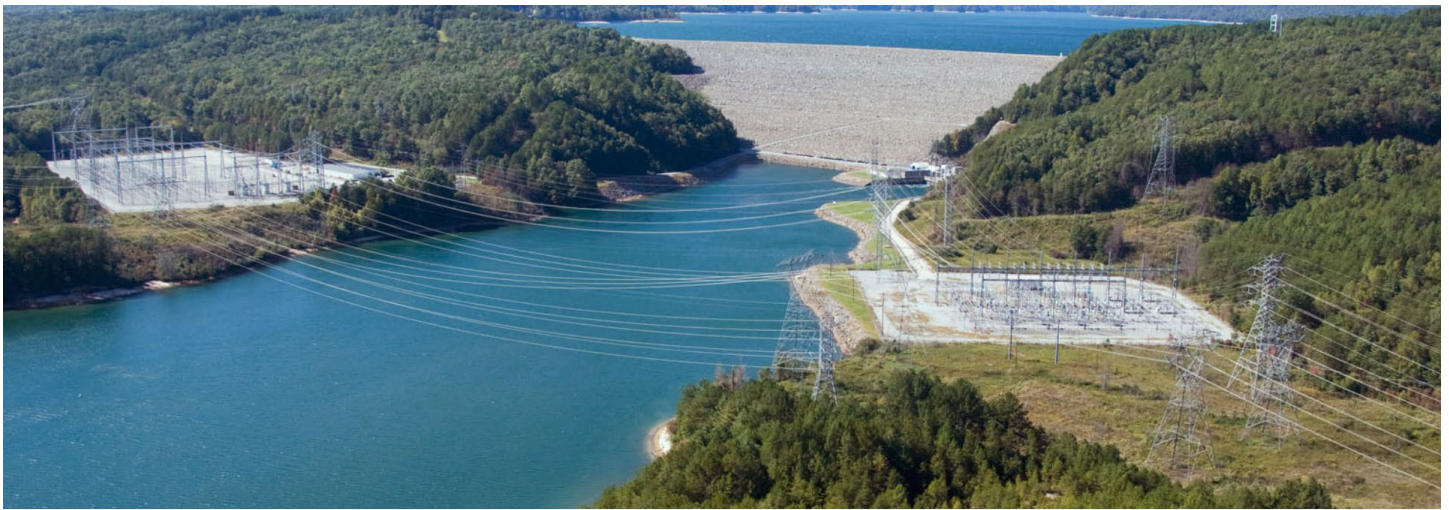
Known as The Marvel in the Mountain, South Carolina's Bad Creek Hydroelectric Station started operating in 1991. The pumped storage hydropower plant can hold up to 1,065 megawatts of renewable energy. Photo courtesy of the National Hydropower Association
