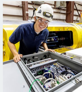
Andrew Simms smiles as he stands over the SeaRAY autonomous offshore power system's Modular Ocean Data Acquisition system, which he and other National Renewable Energy Laboratory researchers built to give remote operators the ability to control the SeaRAY device and receive data from the vehicles it powers. Photo courtesy of the National Renewable Energy Laboratory
