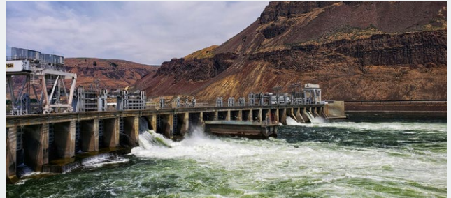
Pumped storage hydropower facilities can store huge amounts of clean energy and help ease the nation's transition to a renewable energy grid. A report lays out this and many more benefits of this valuable form of hydropower. Photo courtesy of Karl Specht, U.S. Department of Energy's Make a Splash Photo Contest
