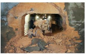
U1a dual-headed mining breakthrough: Two mining crews working over 960 feet underground finish tunneling toward each other to meet in the middle.
