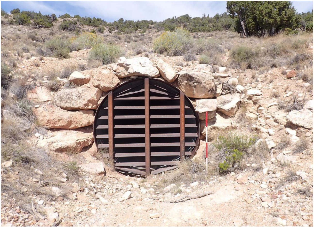
Figure 10. Adit safeguarded with bat-accessible grate (Marie Incline, Mine ID 6021 – Black Hills & Northern Rockies Field Operations Plan).
