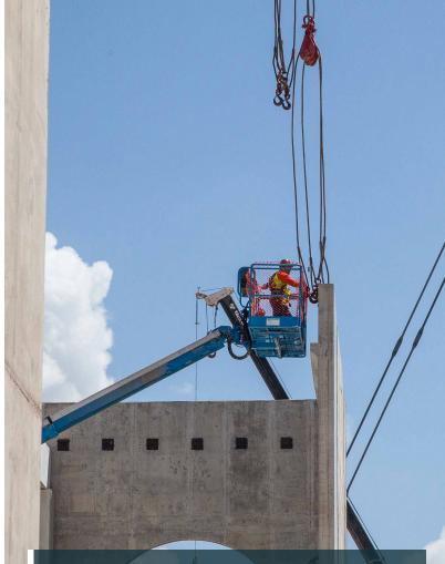
A worker at the Waste Isolation Pilot Plant's Salt Reduction Building locks a precast concrete wall into place.
