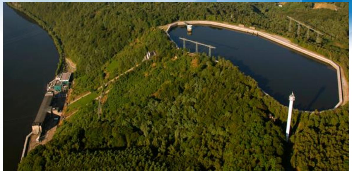
Pumped Hydro Storage – water pumps and power turbines with elevated water storage. Expected lifetime of 30-50+ years.
