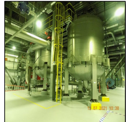
IWTU mercury adsorber vessels
