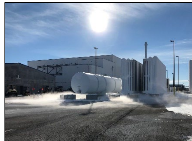
IWTU liquid nitrogen storage system
