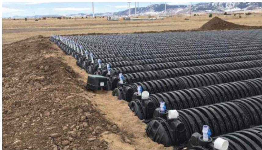
Figure 3.13-2. New Wastewater Treatment System at the FC
