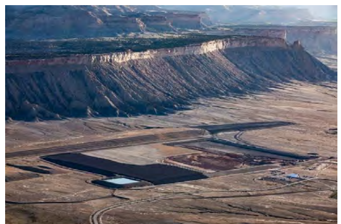
The Crescent Junction disposal cell, about 30 miles away from the Moab Site.
