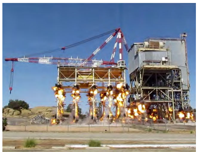
ETEC's final building for demolition – the Sodium Pump Test Facility – amid blasts from shaped charges.
