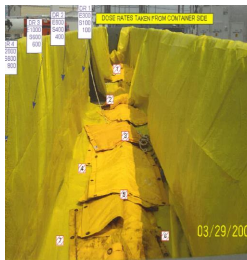
Fig. 4. Exterior of B-36 Disposal Container and Actual Tank 28F Salt Sampling Drill String and Lead Blankets in B-36 Box
