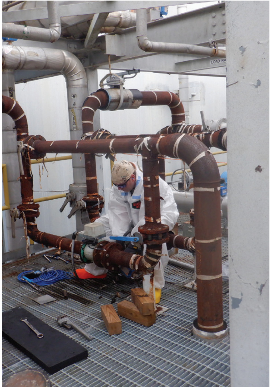
Piping replacement in the 3608 Building
