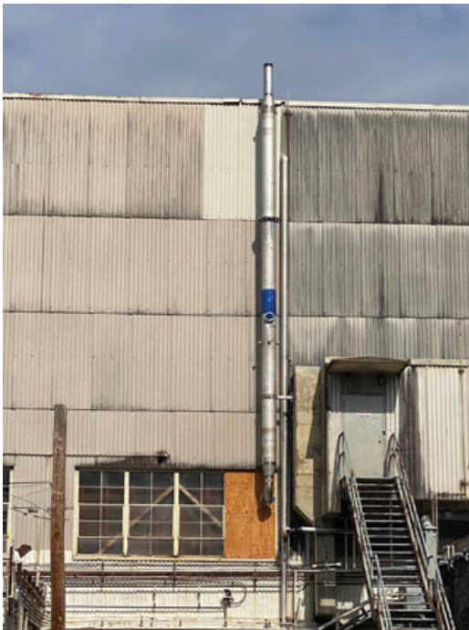
Stack installation for the Continuous Purge System at MSRE
