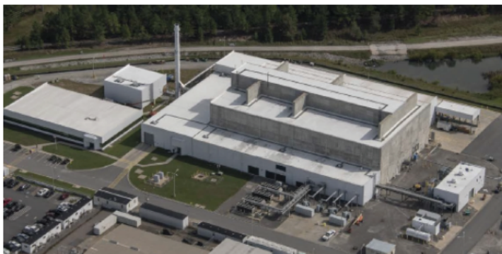
An aerial view of the Salt Waste Processing Facility at the Savannah River Site.
