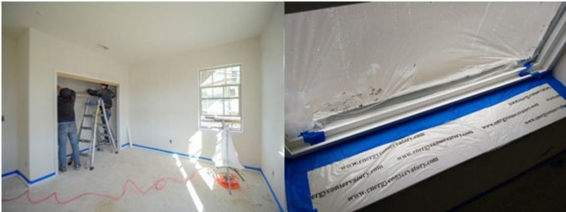
Figure 24. Additional preparation required in Houses #9, #10, and #11 to protect installed trim, including baseboards and shelves (left) and windowsills (right)
