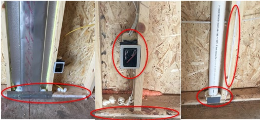
Figure 31. Typical air sealing details: can foam around bottom plate duct and electrical penetration (left), airtight electric box at exterior wall and caulk bottom plate/subfloor (middle), and can foam at plumbing penetration and caulk between framing
