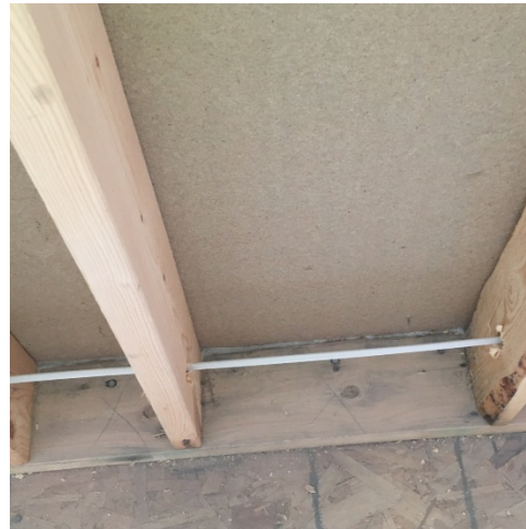
Right: Wall cavities exposed to allow aerosol to seal gaps between sheathing and sill plate
