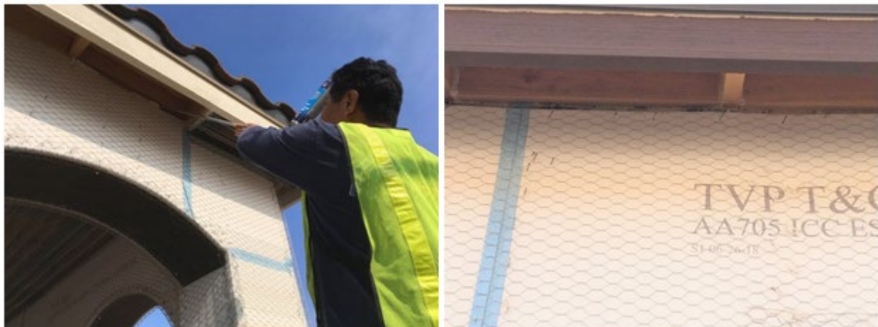
Figure 16. Large gaps at eaves between foam and roof structure were sealed prior to aerosol sealing
