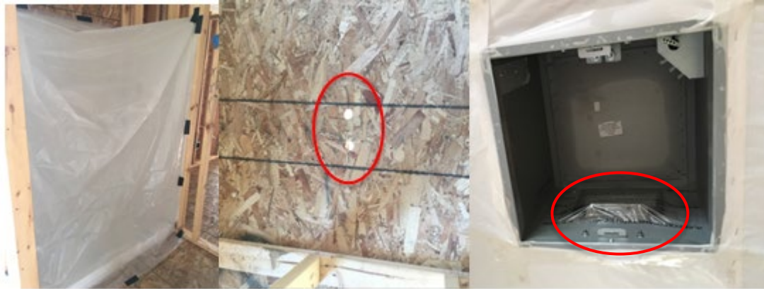
Figure 32. Temporary sealing preparations: shower base, 1-in. holes in subfloor over garage, and exhaust fan outlet
