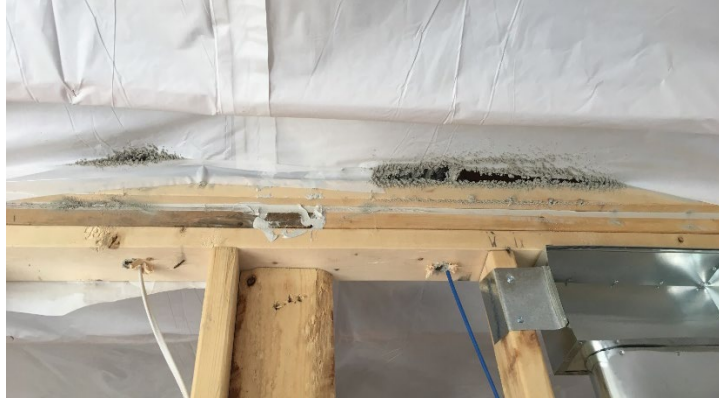
Wrong: Poly sheet pulled away from framing during sealing due to poor stapling and caulking
