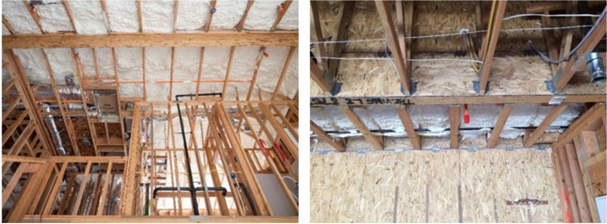
Figure 11. Photos of homes sealed under Option A showing open-cell spray foam at roof deck (left) and rim joist (right)
