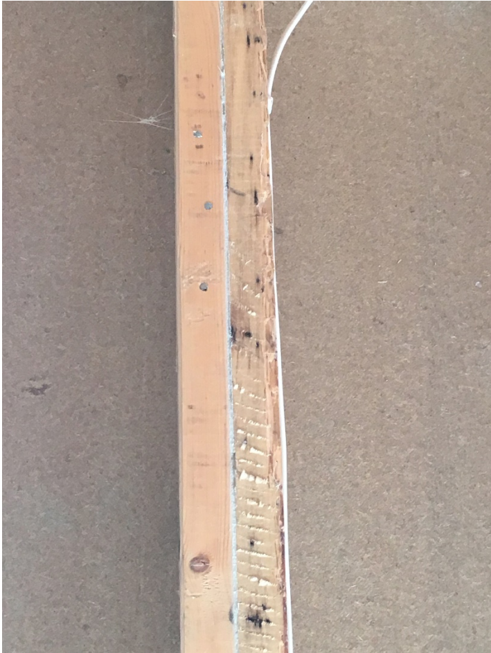
Figure 74. Seal gap between framing
