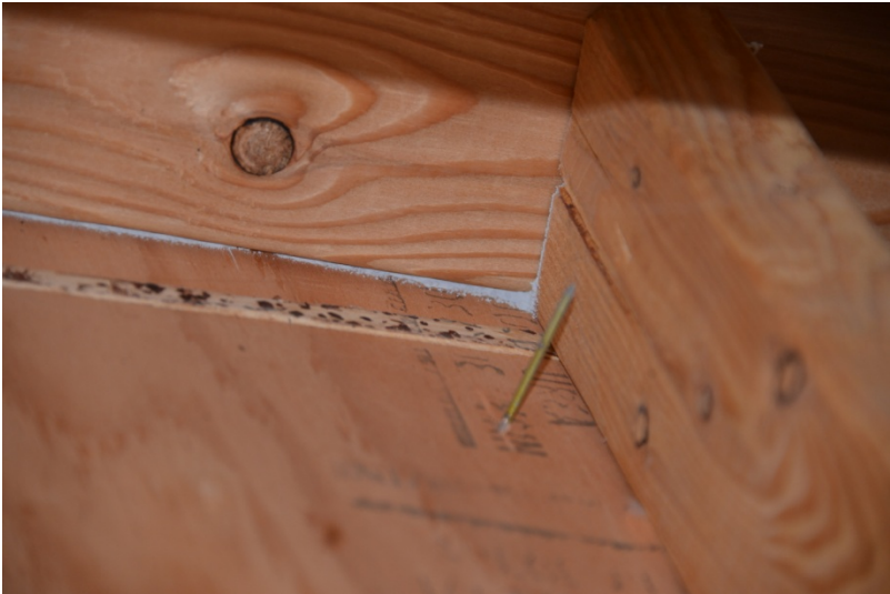
Figure 75. Seal between sheathing and framing
