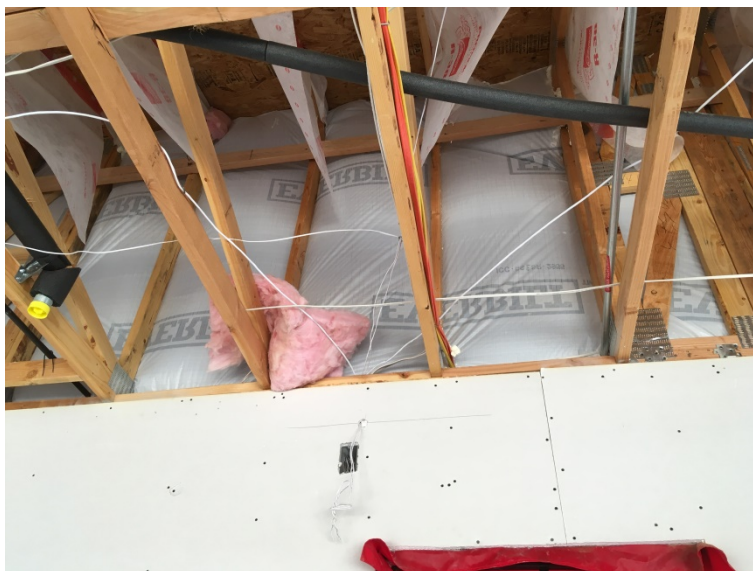
Figure 18. Air barrier wrap above drywall to seal house attic from garage attic
