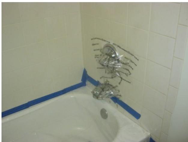
Figure 69. Temporary cover over tub and plumbing fixture
