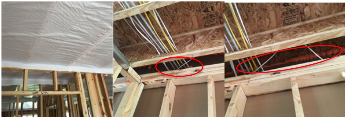
Figure 33. Manual sealing prior to aerosol: poly on second floor ceiling, foam at electrical penetrations to garage, and foam gap at top of garage drywall
