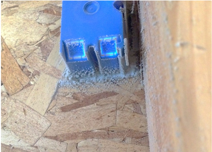
Figure 71. Seal around electric box on exterior wall
