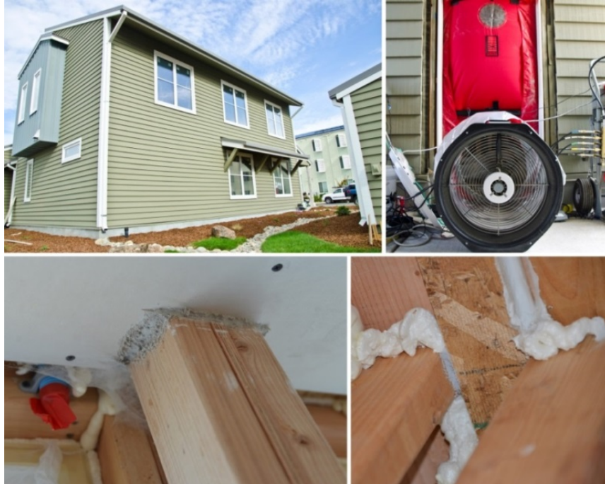
Figure 6. Photos of aerosol sealing installation on a single-family home, including examples of seals formed The contractor was asked to use standard methods to seal leaks with a gap width greater than 0.25 in. (smallest dimension), because the time required to aerosol seal a leak has been shown to increase with the square of the smallest dimension (length or width) of the leak (e.g., it takes four times longer to seal a leak that is 0.5 in. across than to seal a leak that is 0.25 in. across). Figure 7 summarizes the results of the demonstration, highlighting the three discrete phases in the sealing process. The first aerosol sealing application used an airless nozzle injection system with five injection points and without any temperature/humidity control. This injection reduced the building leakage from 4.2 ACH 50 to 2.6 ACH 50 . After the first application, three contractors spent 24 person-hours attempting to further seal the building manually with expanding foam and caulk, resulting in an almost negligible impact on the overall tightness of the building shell. Finally, the aerosol envelope sealing process was applied again, this time using air-atomization nozzles and temperature/humidity control. That process reduced the building leakage from 2.6 ACH 50 to 0.8 ACH 50 in about 4 hours of total injection time. In summary, the Honda Smart Home demonstration revealed the advantage of using the aerosol envelope sealing process over standard manual sealing methods. Relying on manual sealing to accomplish the level of airtightness desired would have required a substantial amount of time and labor.
