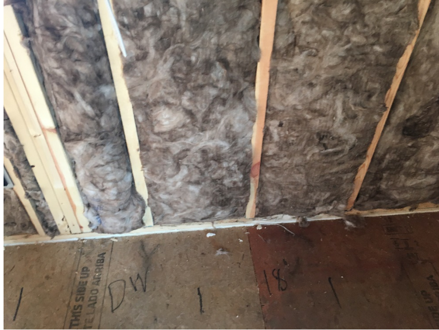
Wrong: Batt insulation installed prior to aerosol sealing at early phase of construction
