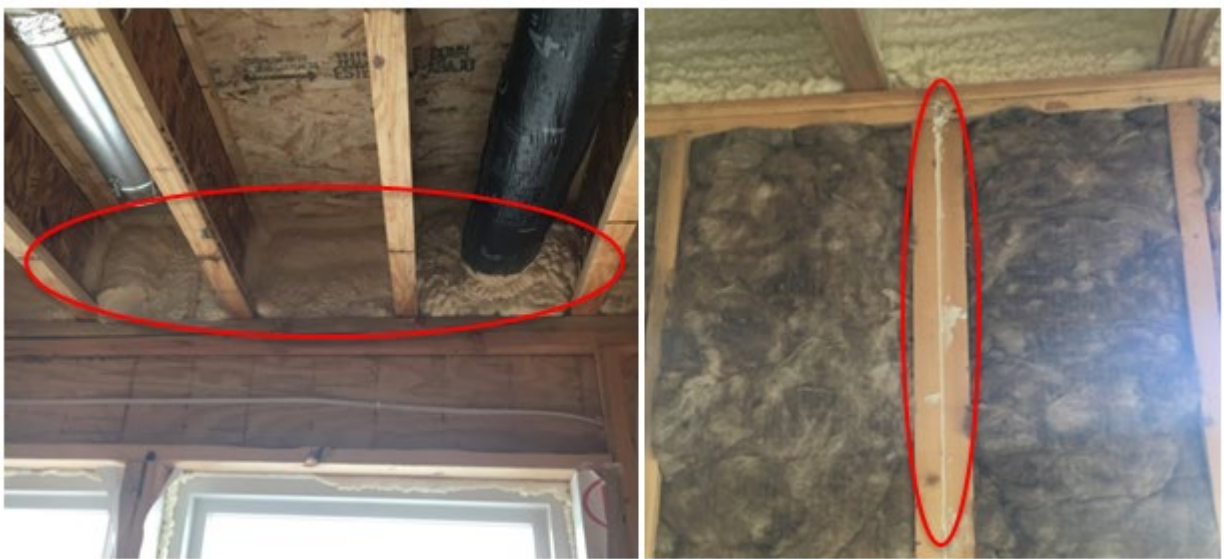
Figure 28. Closed-cell spray foam at rim joist and duct penetrations (left); caulk at seams where wood is joined (right)
