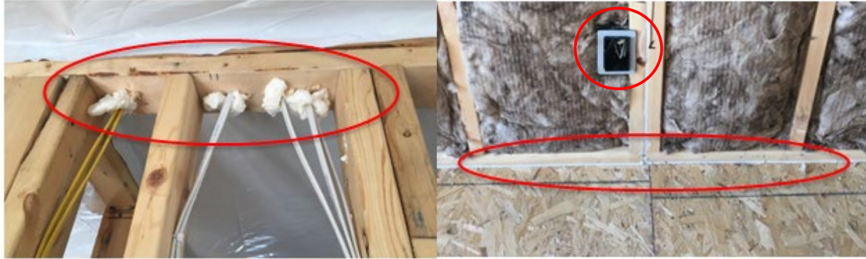
Figure 29. Can foam at wire penetrations (left); foam gasket/caulk at sill plate and airtight electric box (right)
