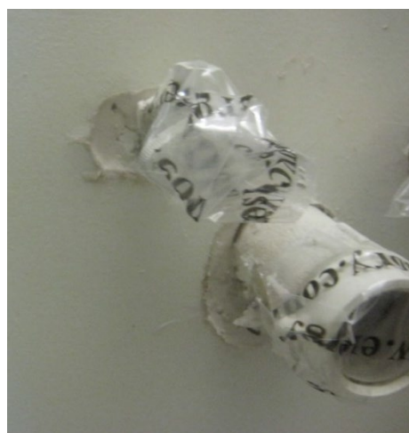
Figure 68. Temporary cover over open plumbing pipes
