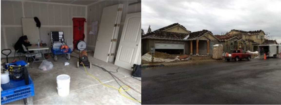
Figure 23. Aerosol equipment set up in garage with kerosene heater (left); Houses #10 and #11 sealed during rain (right)
