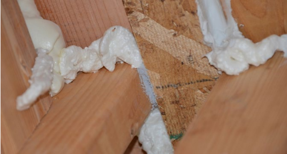
Figure 70. Seal (gray material) formed between gap in foam
