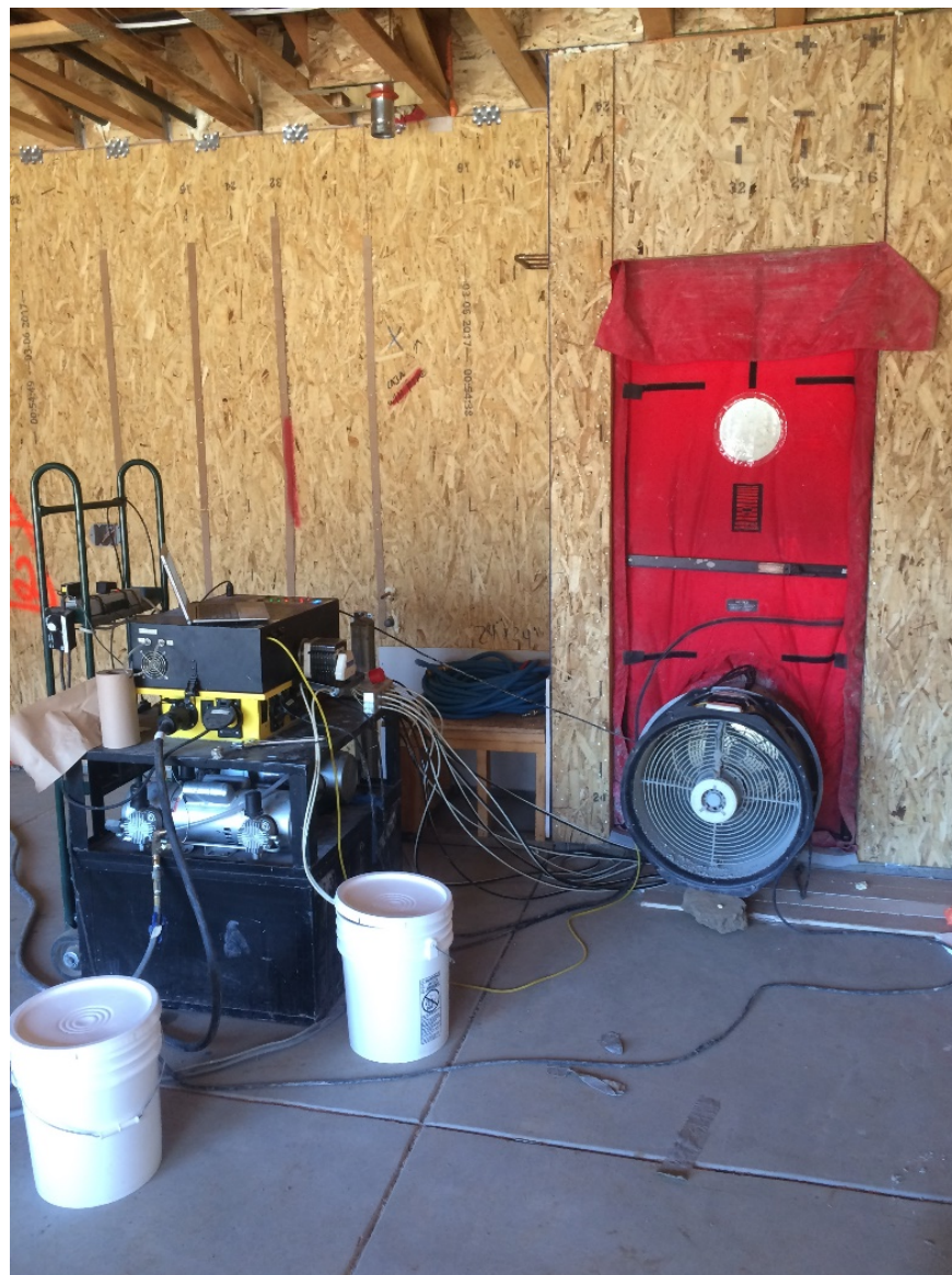
Figure 66. Blower door, sealant pump, and sealant setup in attached garage
