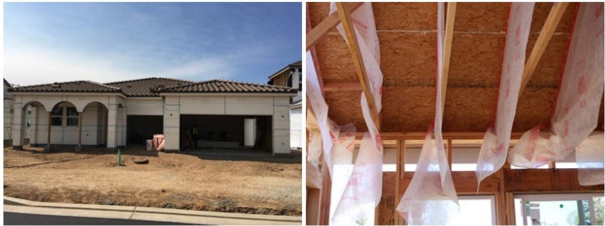
Figure 17. Bibs attached to roof deck left hanging (left); photo of home sealed with ridged foam on exterior (right)
