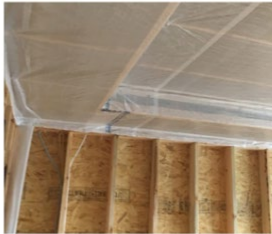
Right: Poly sheet properly stapled and caulked for aerosol sealing at early phase of construction; a high level of care is required for the poly to hold up to the high pressurization (100 Pa) that occurs during sealing
