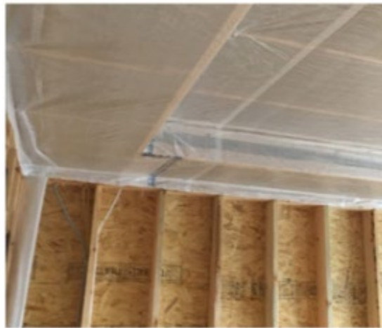
Figure 30. Interior poly sheet on top floor ceilings and exterior walls
