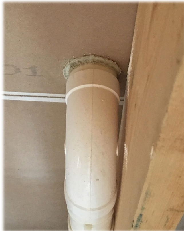
Figure 73. Seal between plumbing penetration and drywall
