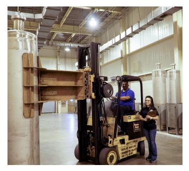
Workers use a special forklift to move an empty canister for its inspection at DWPF. The canister will be filled with vitrified high-level waste.
