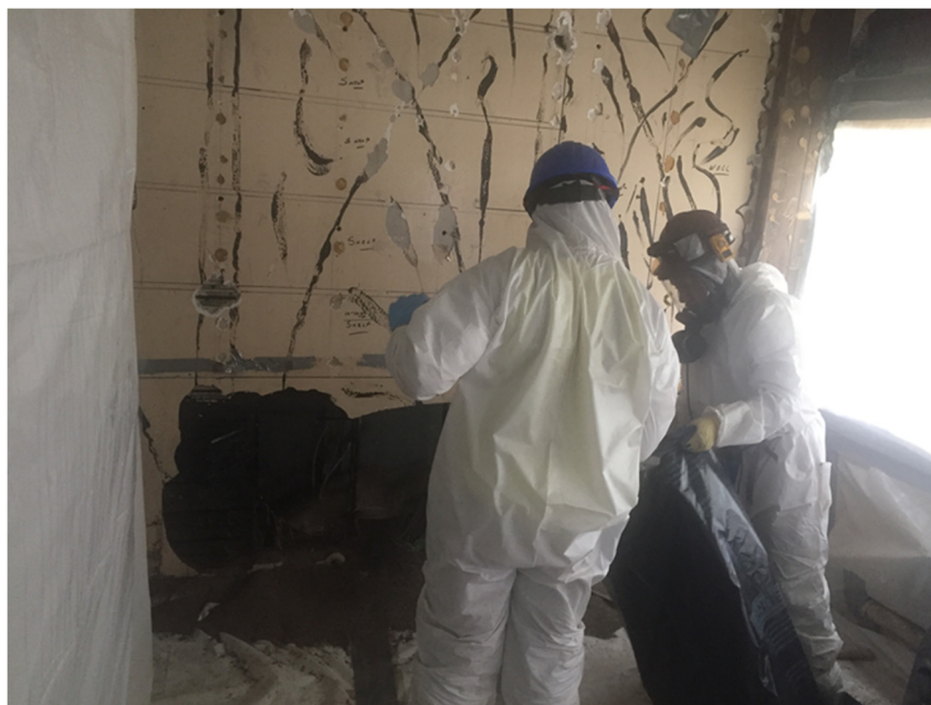
Photo 8. Asbestos Workers Removing Vermiculite for Disposal
