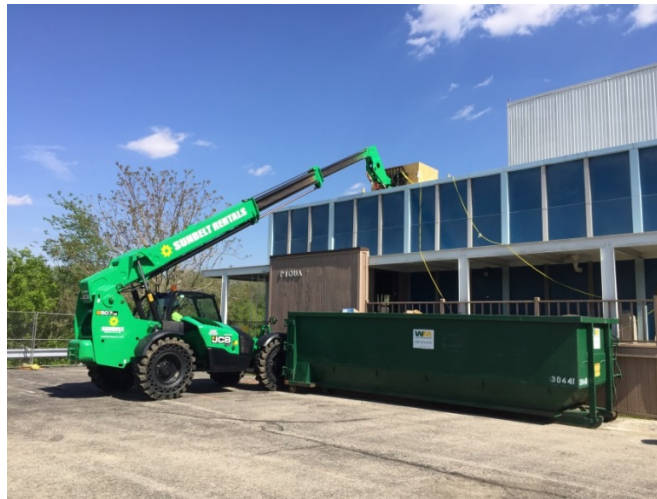
Photo 6. Using a Telehandler to Move the Waste Box
