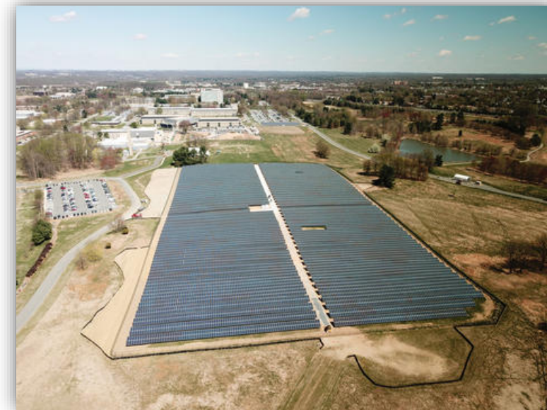
National Institute of Standards and Technology (NIST) 5 MW-DC solar PV array in Gaithersburg, MD. Awarded as an ESPC energy sales agreement under ENABLE. Photo courtesy of NIST
