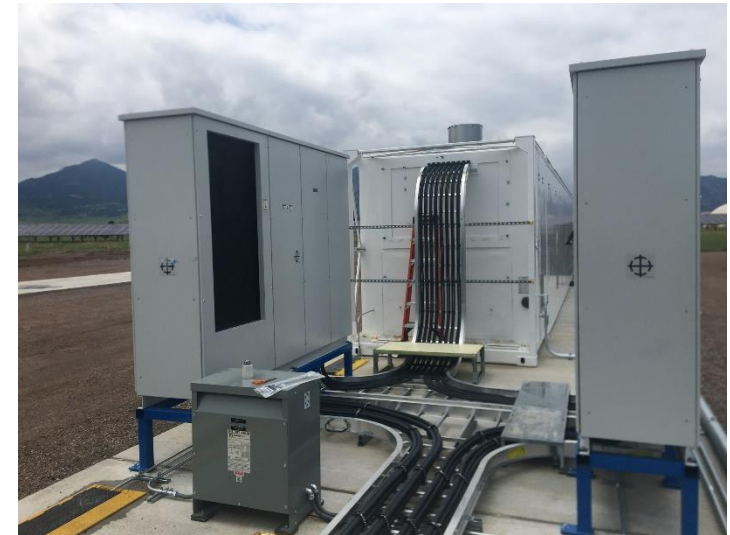
2x1MW GE LV5 Solar inverters
