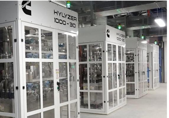
**Air Liquide - Bécancour, Quebec** 4 x HyLYZER® 1000-30 – indoor – 20 MW – 8,000 kg/day WORLD'S FIRST HYDROGEN REFUELING STATION CAPABLE OF SUPPLYING GREEN HYDROGEN DIRECTLY TO SHIPS, CARS, TRUCKS AND INDUSTRIAL CUSTOMERS
