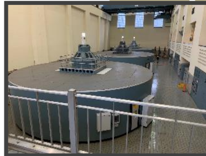
Center Hill Turbine-Generator Rehab
