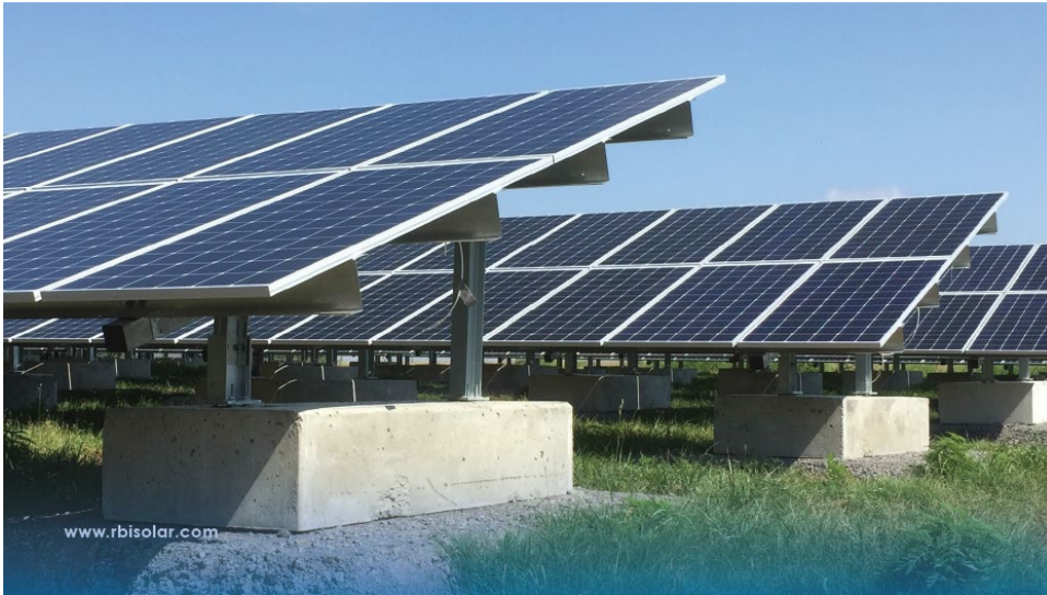
Concrete ballast mounted PV panels
