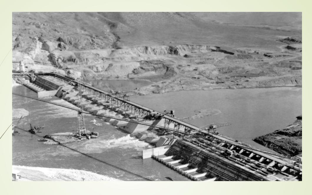
Grand Coulee Dam is a concrete gravity dam on the Columbia River in the U.S. state of Washington, built to produce hydroelectric power and provide irrigation water. Constructed between 1933 and 1942
