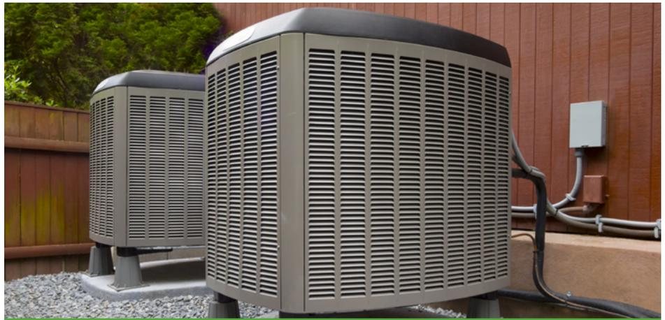
Cold-climate heat pumps (CCHPs) provide both space heating and cooling for homes, and incorporate advanced features that allow for improved heating capacity and efficiency at cold weather conditions compared with traditional heat pumps.
