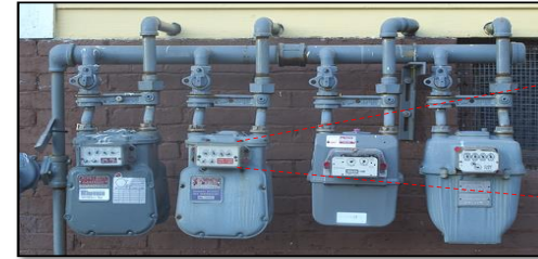
(a) Typical Installation of Diaphragm Natural Gas Meters
