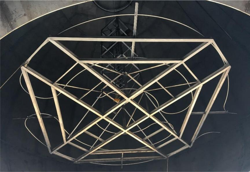
**Top manifold and support tower being lifted into place**
