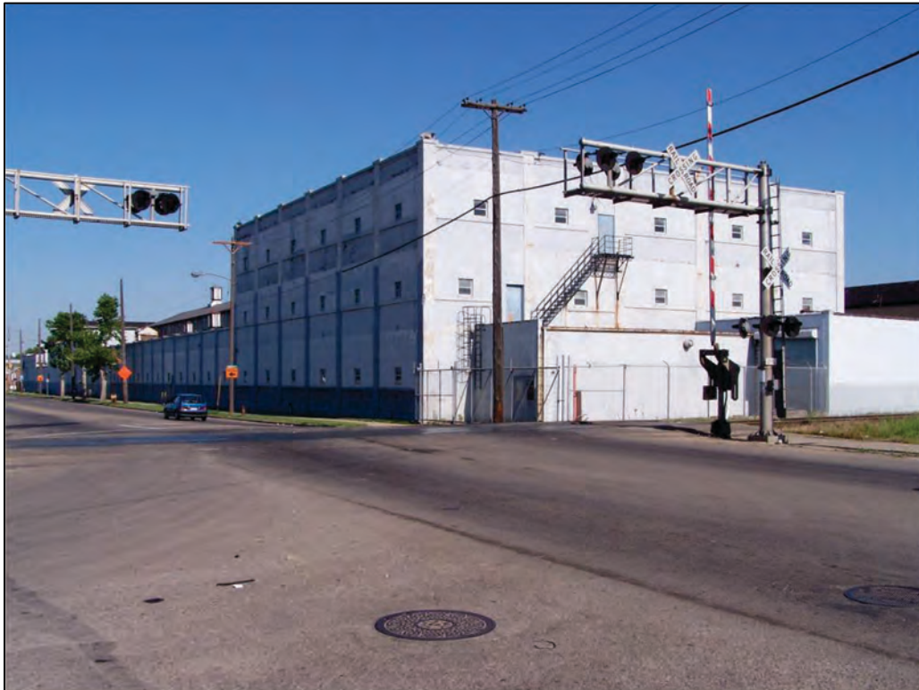
Figure 17-2. Former HHMS Company Building (circa 2006) Showing the Third Floor, Where FUSRAP Remediation Occurred
