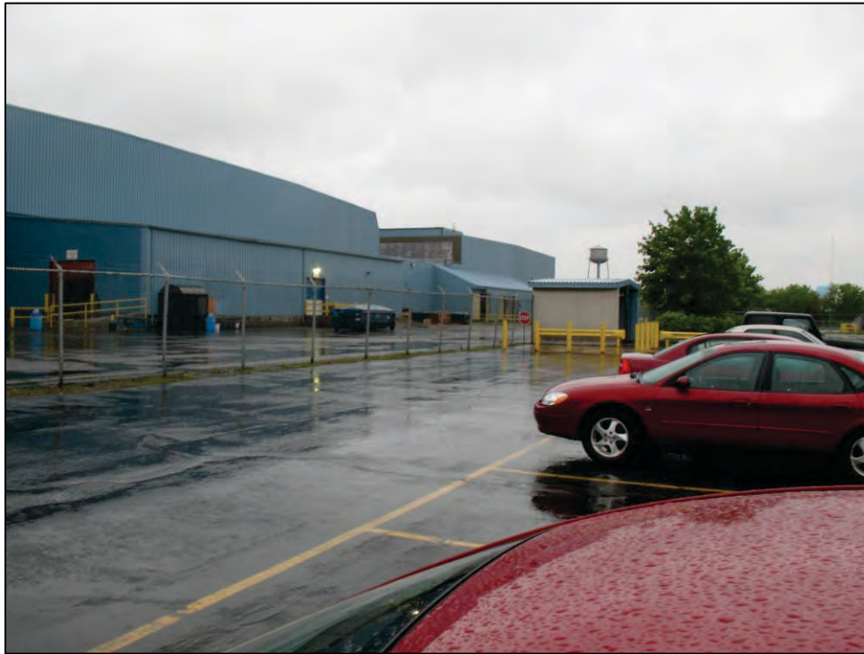
Figure 3-4. Adrian, Michigan, Site, July 2010
