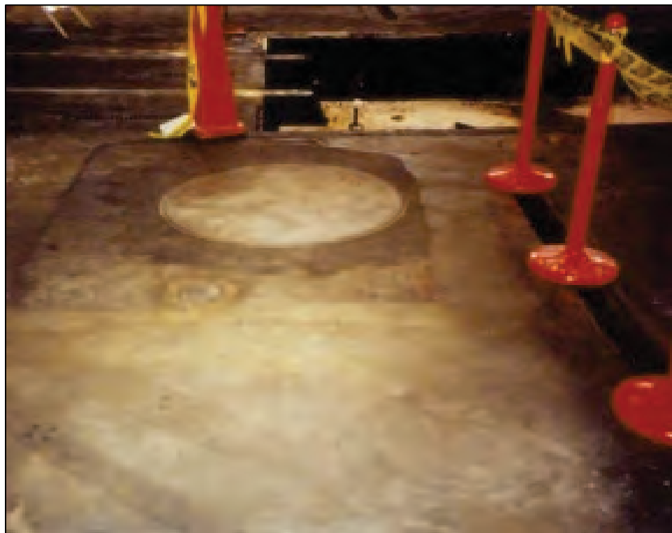
Figure 3-3. Adrian, Michigan, Site Remediated Area, July 1995 (DOE Digital Archive)
