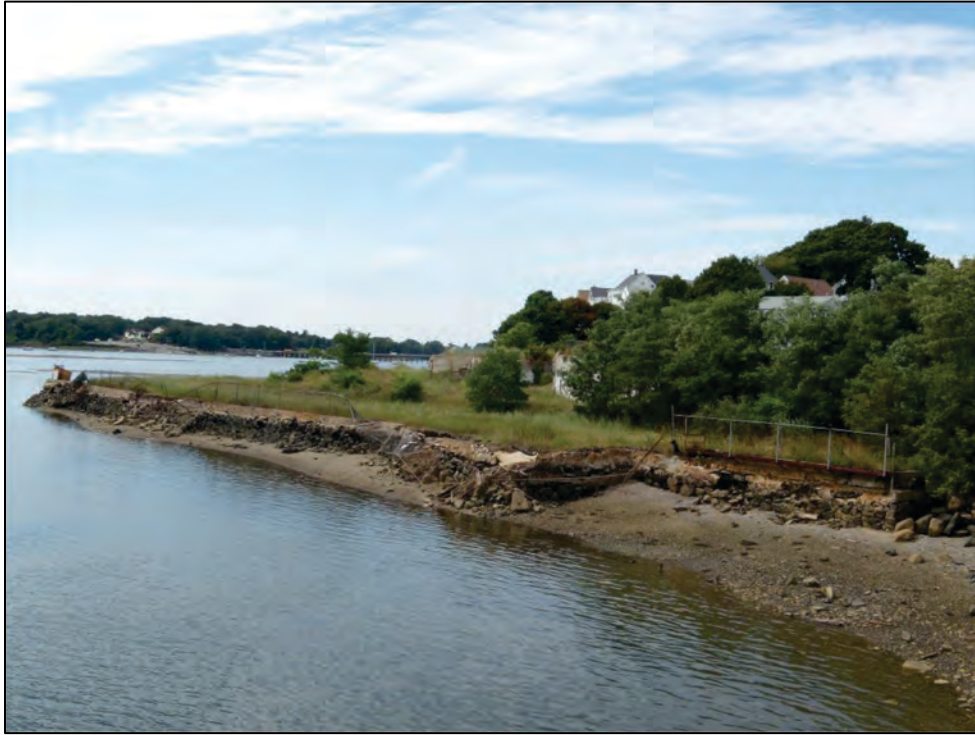
Figure 9-2. Beverly, Massachusetts, Site Looking West from a Railroad Bridge, August 2010
