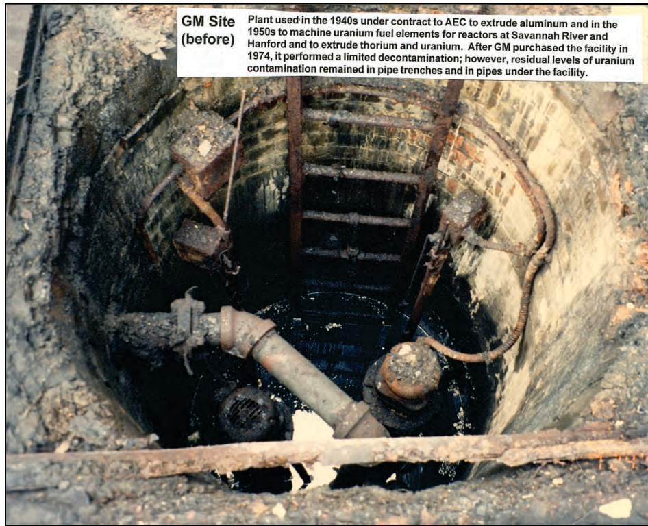
Figure 3-2. Manhole at the Adrian, Michigan, Site Before Remedial Action, December 1974 (DOE Digital Archive)
