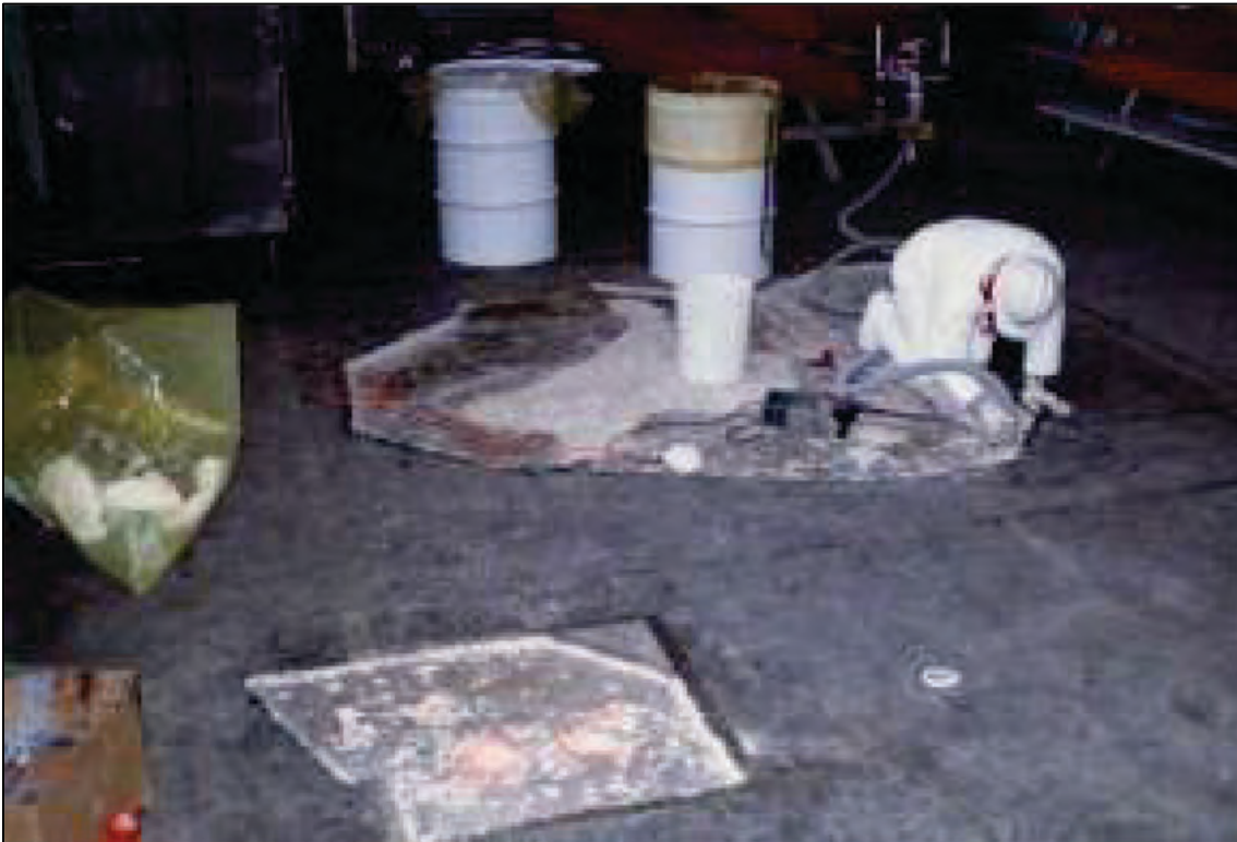
Figure 11-3. Scabbling Concrete at the Chicago North Site, September 1987 (DOE Digital Archive)
