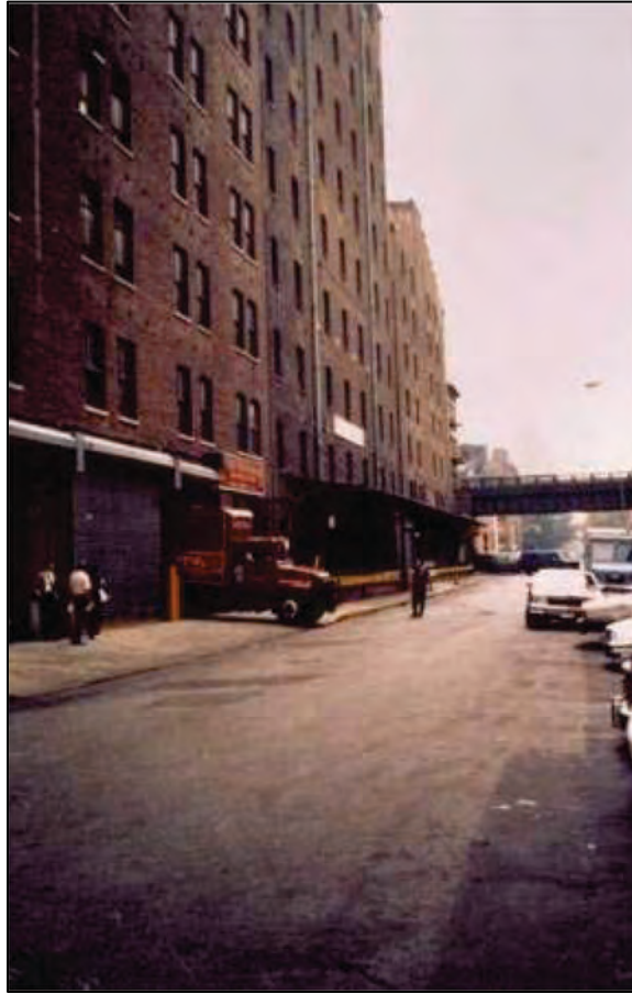
Figure 22-2. Baker and Williams Warehouses, 1990 (DOE Digital Archive)
