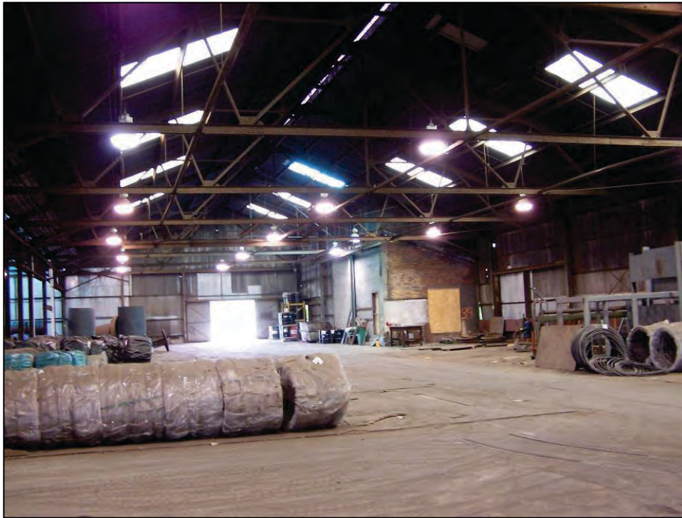
Figure 5-4. Building Interior, Aliquippa, Pennsylvania, Site, September 2005
