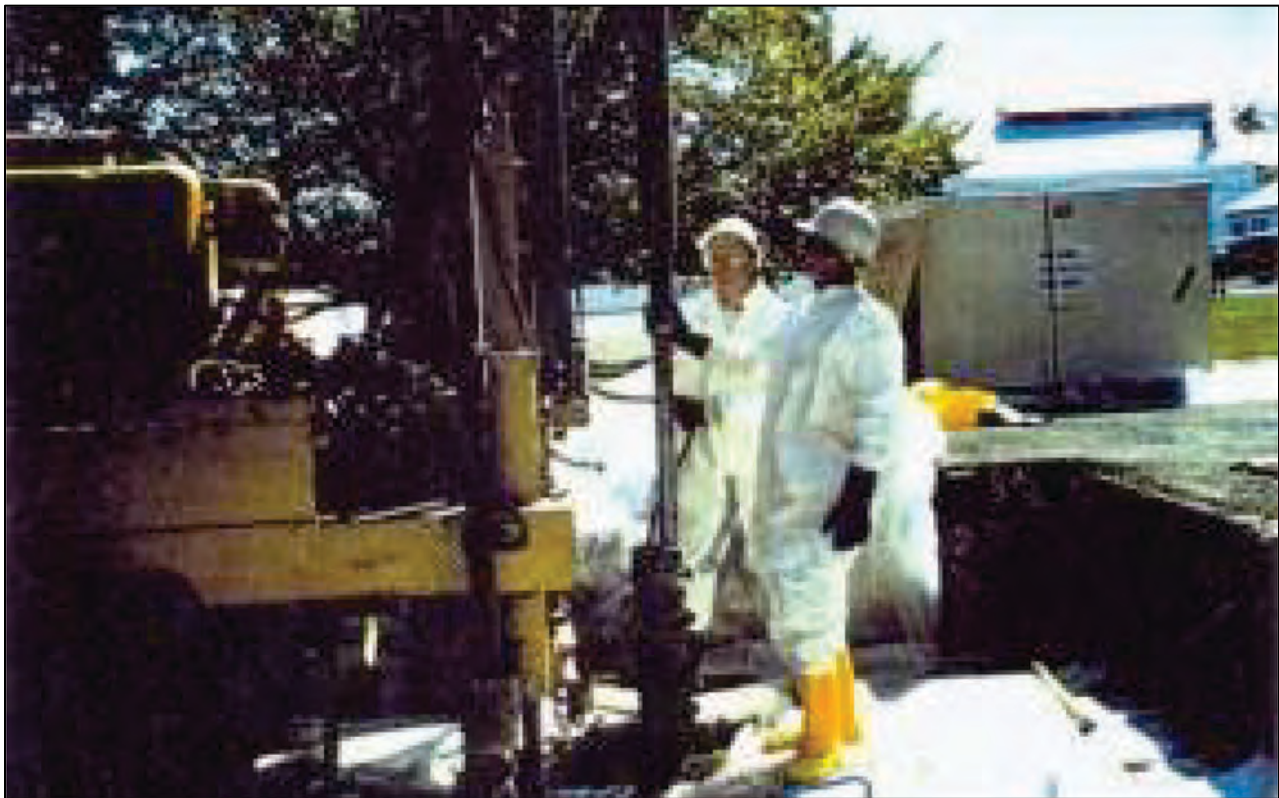
Figure 4-3. Radiological Survey Support Work at the Albany, Oregon, Site, December 31, 1991 (DOE Digital Archive)
