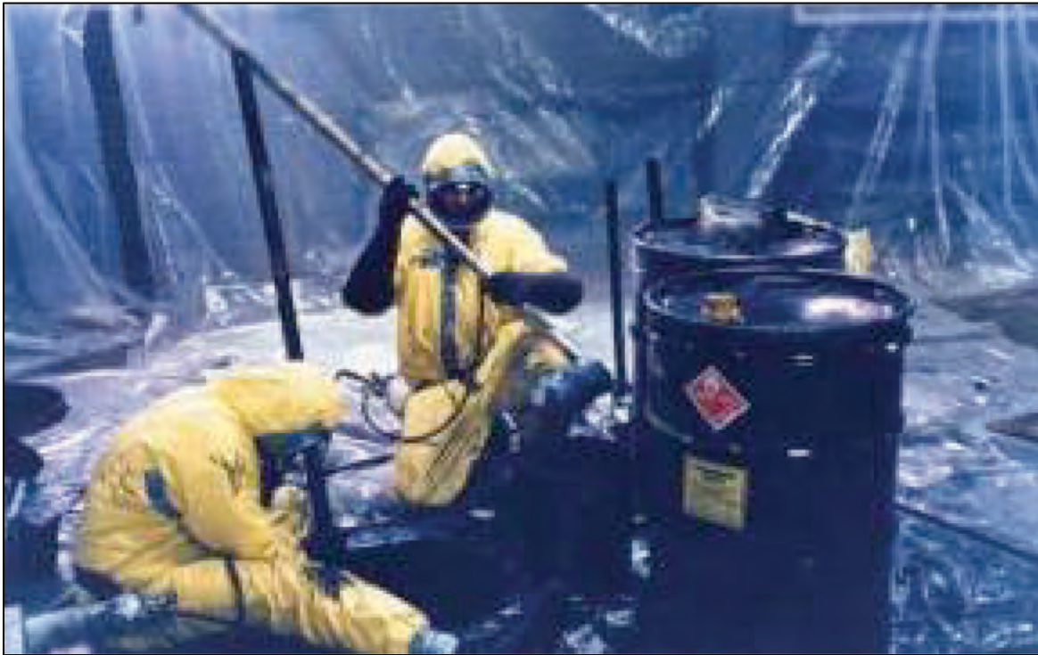
Figure 11-2. Removing Sludge and Placing It in Drums at the Chicago North Site, September 1987 (DOE Digital Archive)
