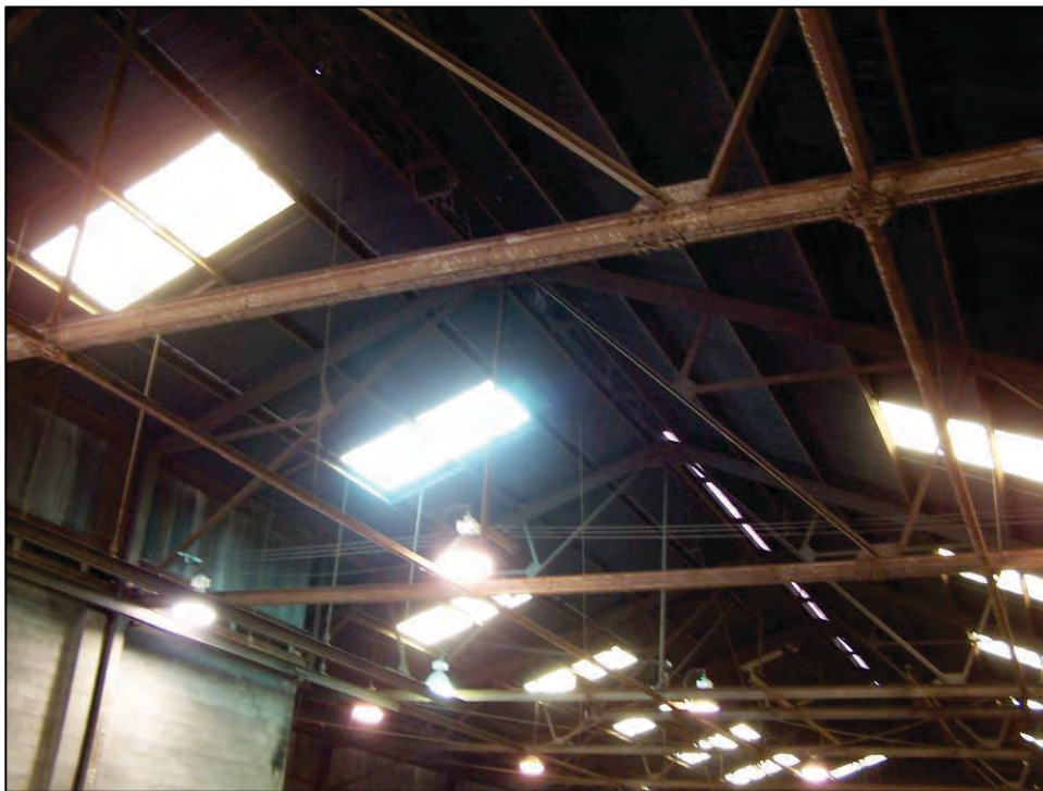
Figure 5-5. Roof System Where Supplemental Limits Were Applied, Aliquippa, Pennsylvania, Site, September 2005
