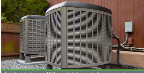
Cold-climate heat pumps (CCHPs) provide both space heating and cooling for homes, and incorporate advanced features that allow for improved heating capacity and efficiency at cold weather conditions compared with traditional heat pumps.
