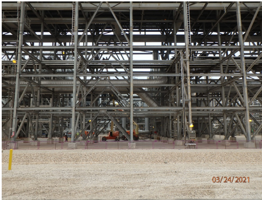
Working punch list items in Train 3 after performance test completed
