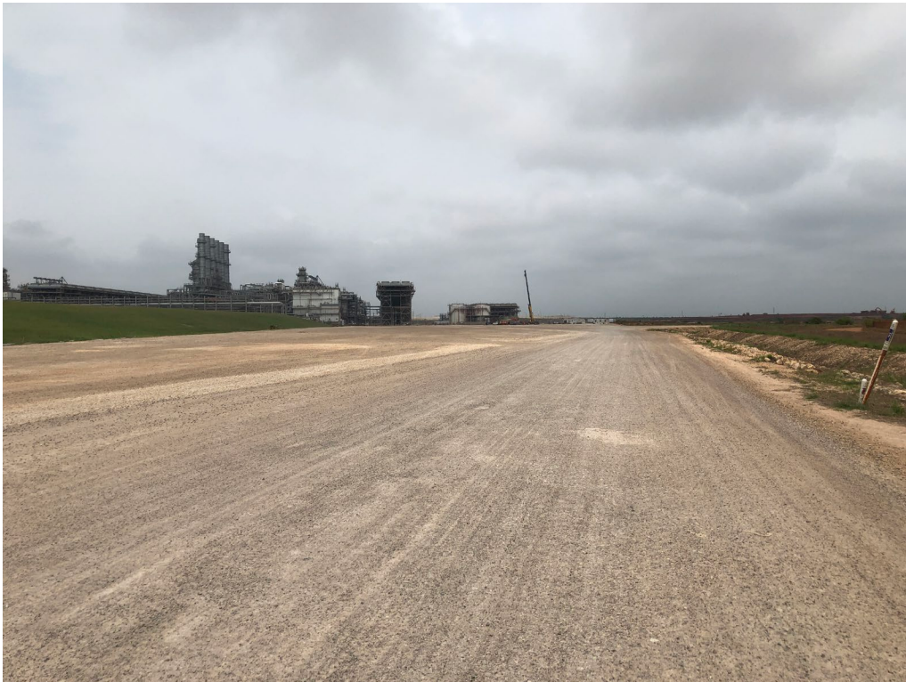
Crushed concrete stablization at Blade Tract. Photo taken April 13, 2021.
