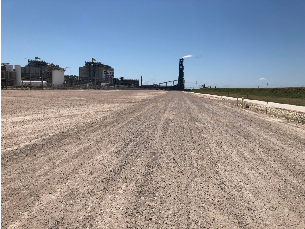
Crushed concrete stablization at 200-Foot Strip. Photo taken April 20, 2021.
