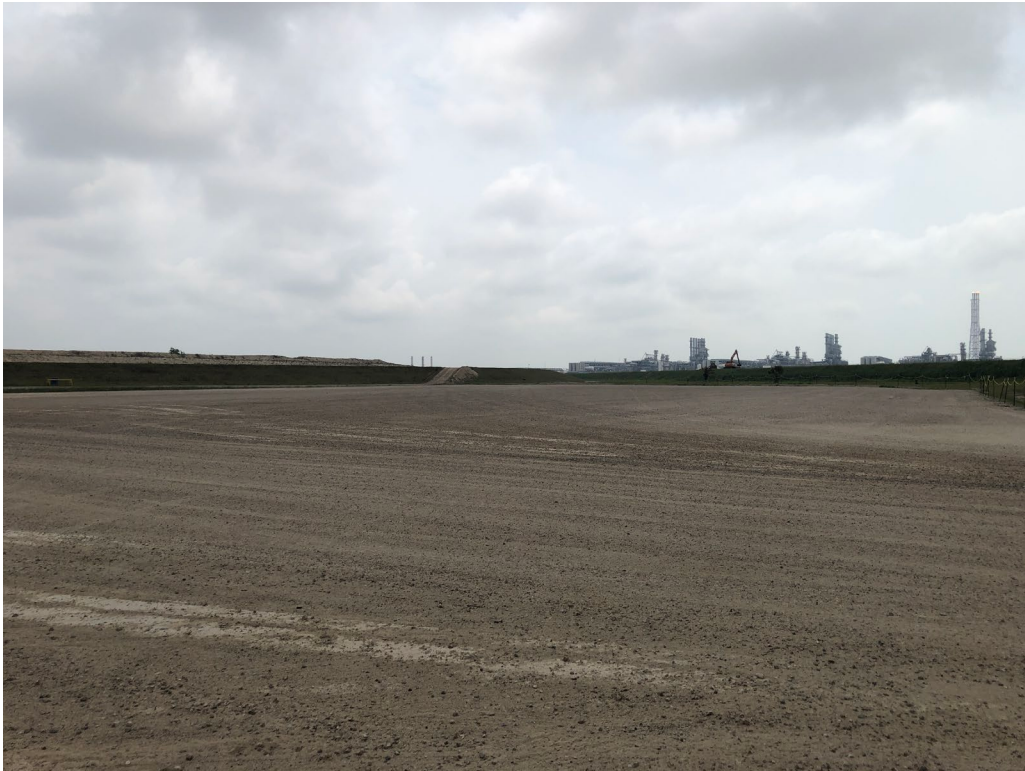
Crushed concrete stabilization at Triangle Area. Photo taken April 13, 2021.
