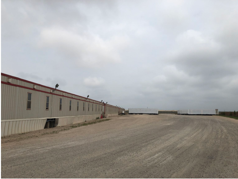
Crushed concrete stablization at Dagger Tract. Temporary office trailers to be removed. Photo taken April 13, 2021.
