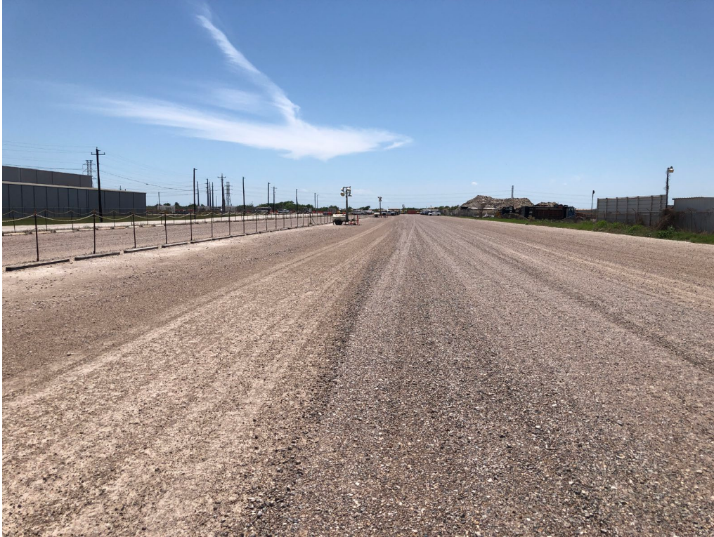
Crushed concrete stablization at Solis 3 Tract. Photo taken April 20, 2021.
