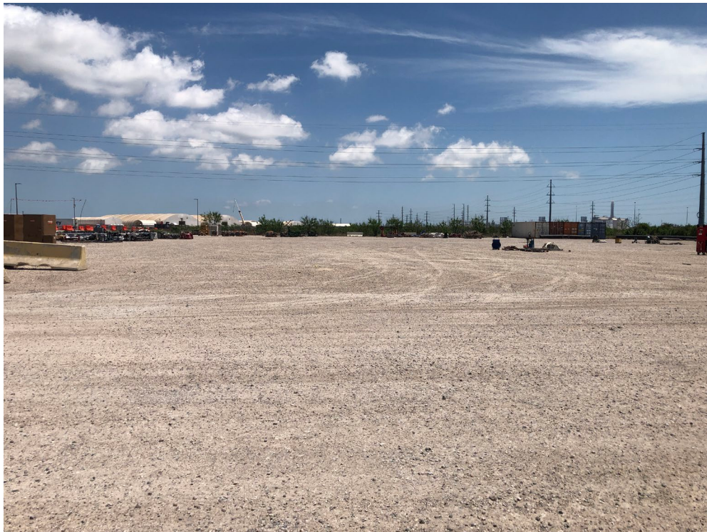
Crushed concrete stablization at Solis 1 Tract. Photo taken April 20, 2021.
