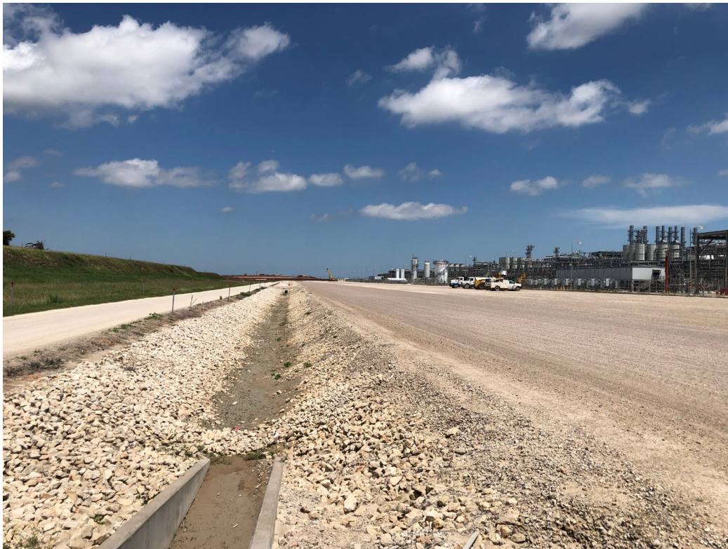
Stablized rock-lined ditch and crushed concrete at 200-Foot Strip. Photo taken April 20, 2021.
