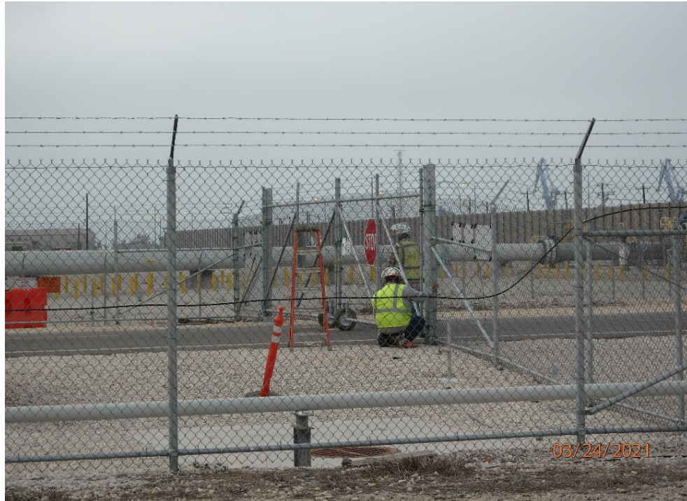
Final fencing and gate work with access control system
