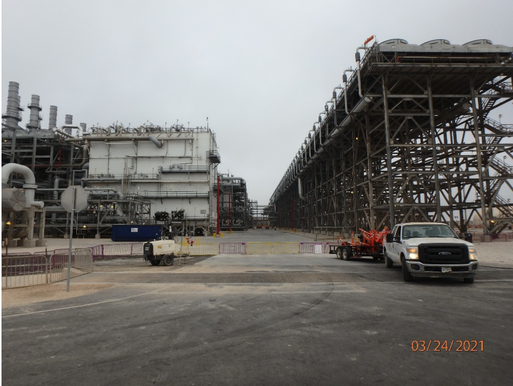
Demobilize temporary facility from Train 3 area
