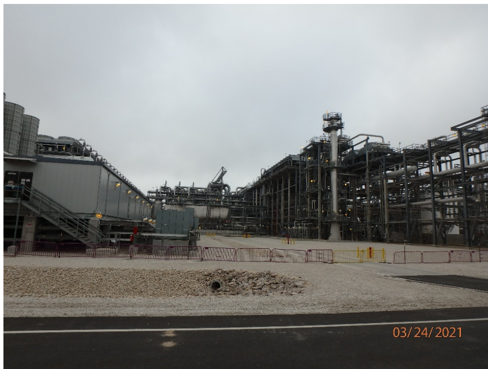
North side of Train 3 area cleared for final turn over
