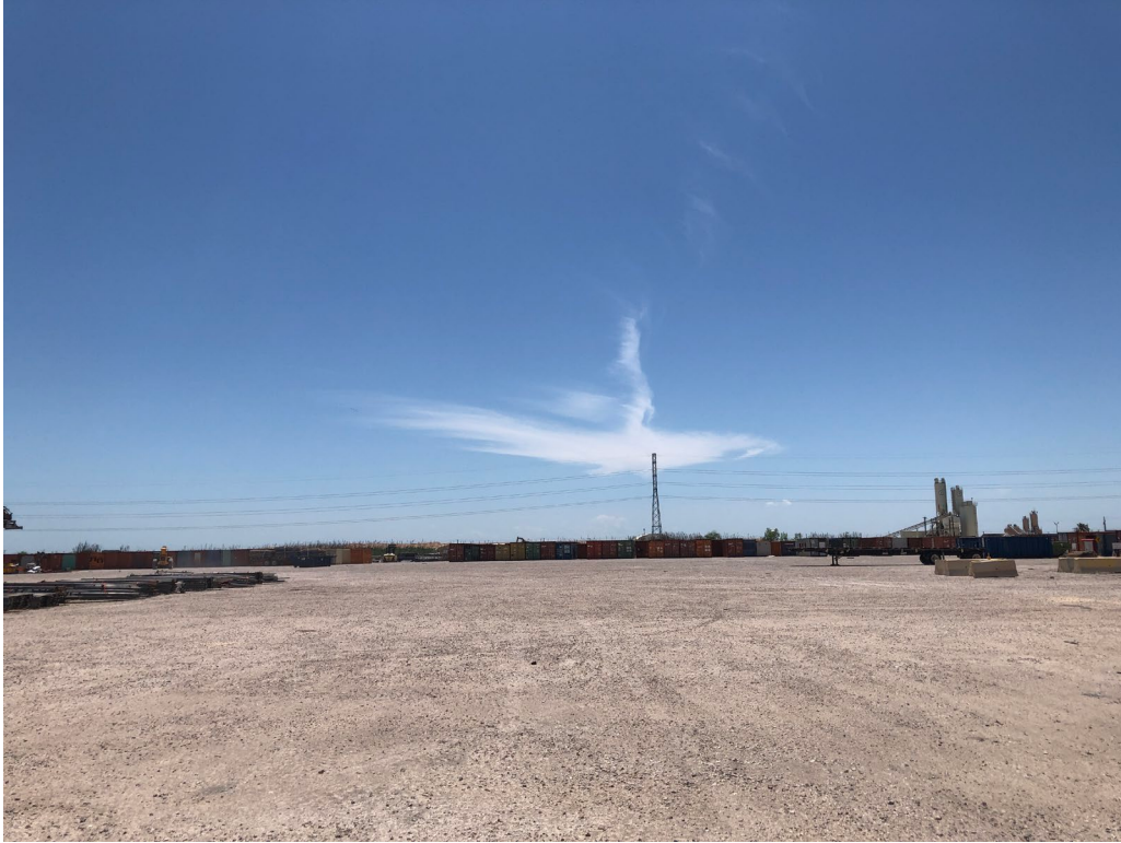
Crushed concrete stablization at Gillespie Tract. Photo taken April 20, 2021.
