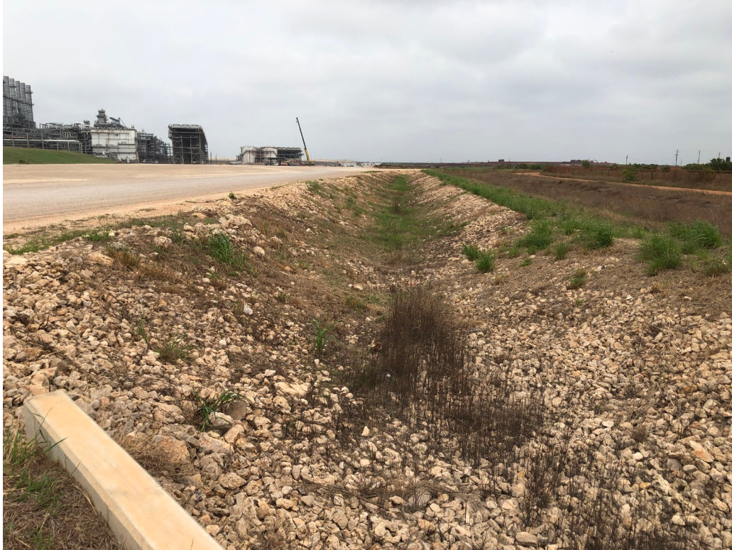
Stablized rock-lined ditch and crushed concrete at Blade Tract. Photo taken April 13, 2021.
