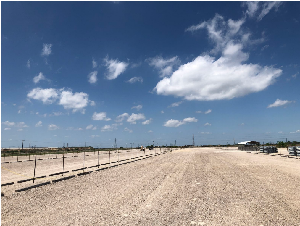
Crushed concrete stablization at Prairie Tract. Photo taken April 20, 2021.
