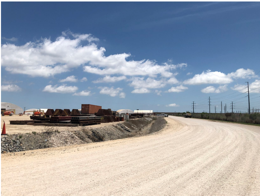
Crushed concrete stablization and rock-lined ditch at Berryman Laydown. Photo taken April 20, 2021.
