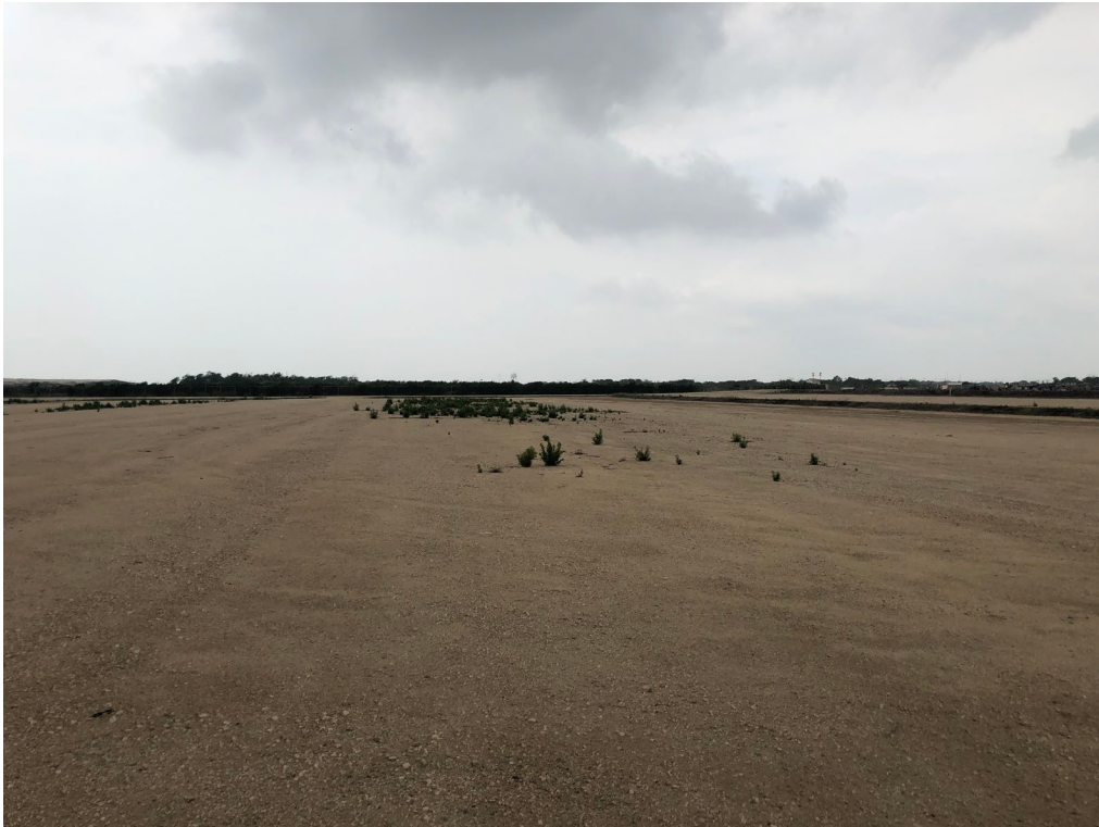
Crushed concrete stablization at 110-acre Port Laydown. Photo taken April 13, 2021.
