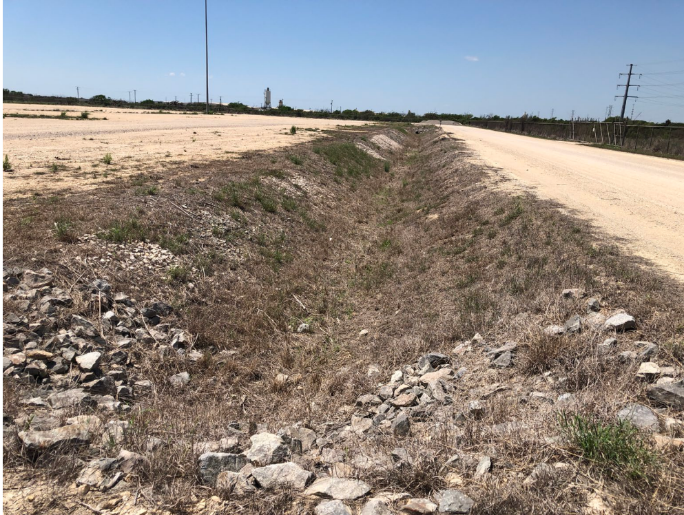
Stablized rock-lined ditch and crushed concrete at 110-acre Port Laydown. Photo taken April 20, 2021.
