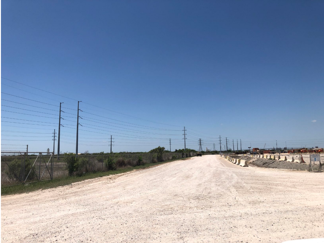
Crushed concrete stablization at Berryman Laydown. Photo taken April 20, 2021.
