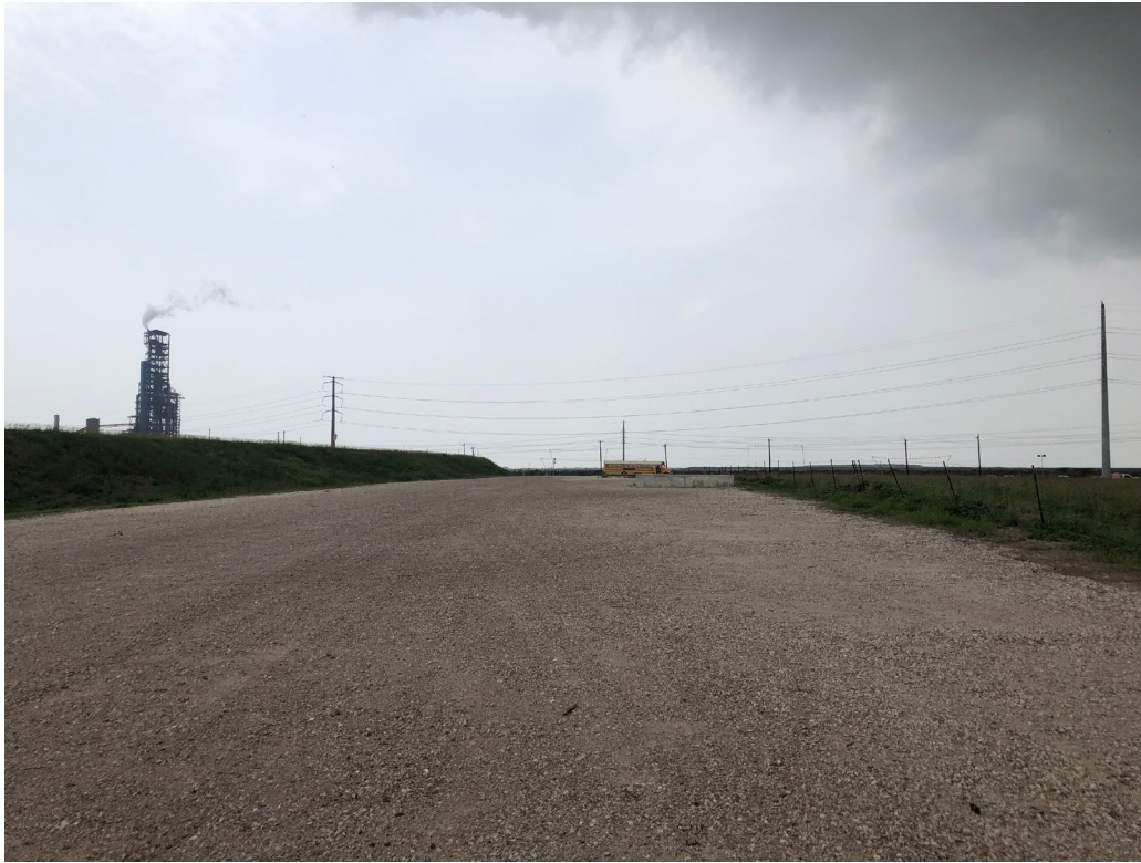
Crushed concrete stablization at Truck Staging Area. Photo taken April 13, 2021.
