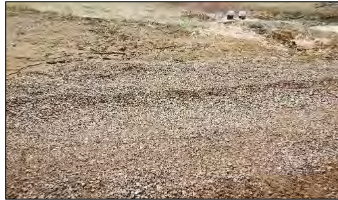
Above East Subsurface Drain Outfall Channel
