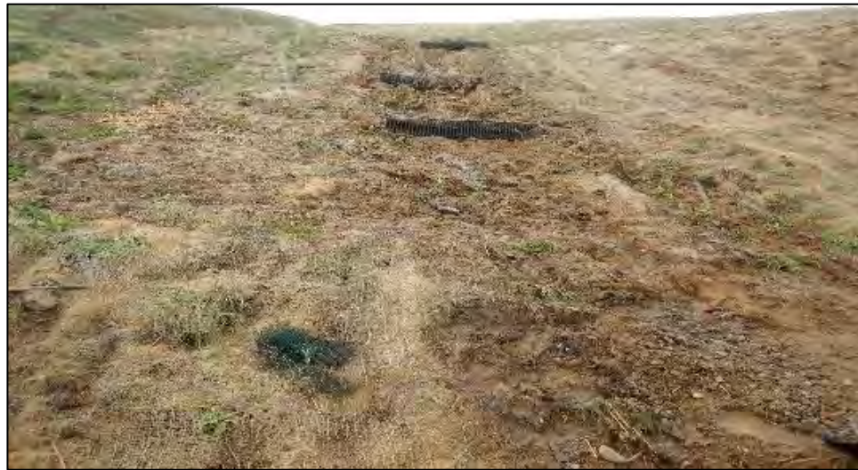
Rills/Gullies in West Perimeter Channel
