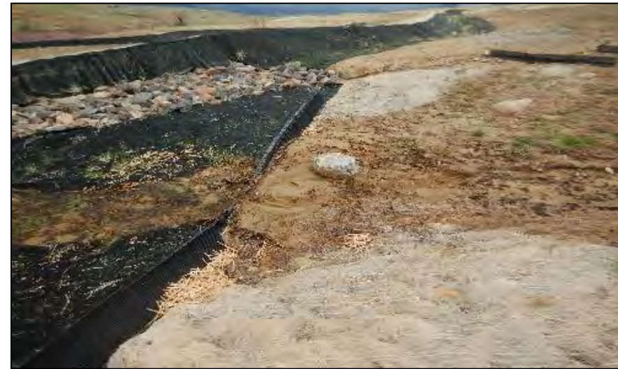
Sediment on East Perimeter Channel GeoRidges
