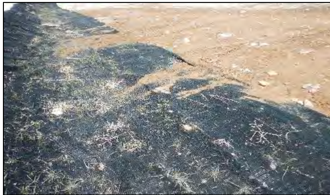
Above Berms 5 and 6
