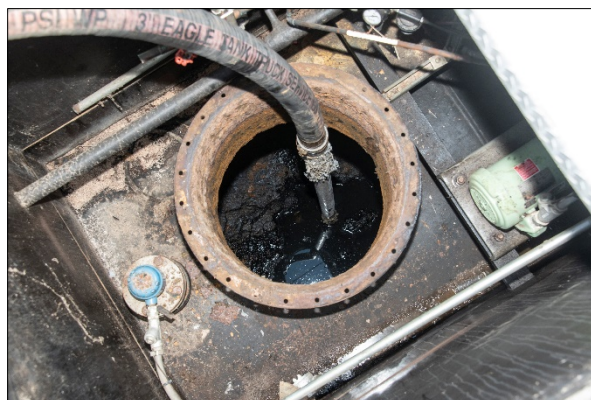
A Special Vacuum-equipped Truck was Used to Remove Water, Exposing a Layer of Sludge Containing Silver to be Recovered.
