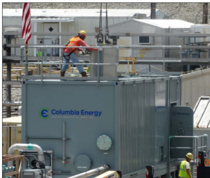
Ion Exchange Column Installed at TCCR
