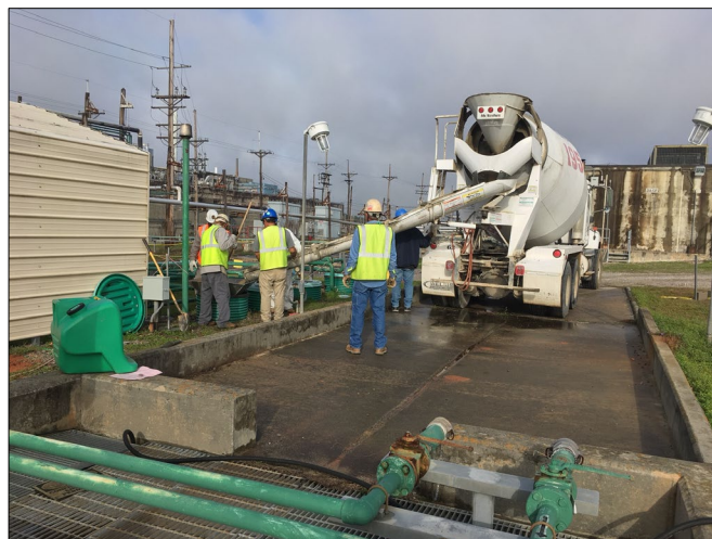
F-Canyon Grouting during F-Canyon UST Closure
