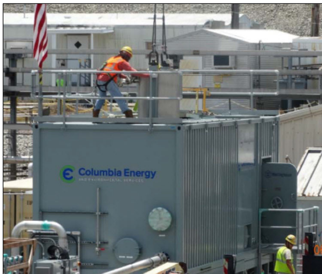
Ion Exchange Column Installed at TCCR
