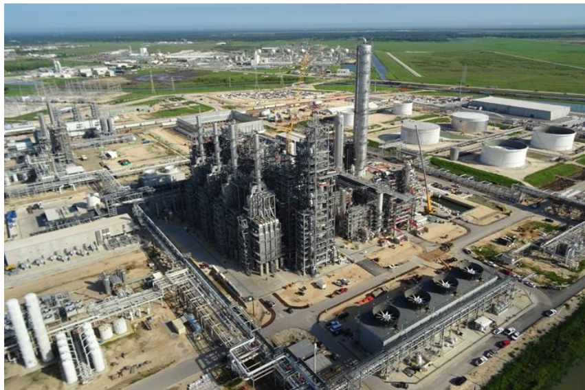
Dow PDH plant Freeport, TX Typical reaction temperature 500-600 °C
