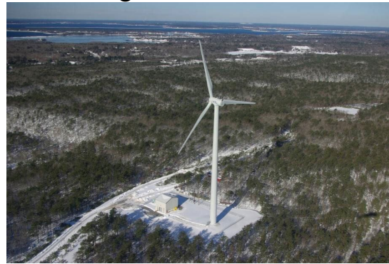
Microgrids can operate connected or disconnected from “the grid.” Joint Base Cape Cod – Otis, Buzzards Bay, MA, USA
