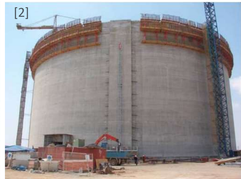
A concrete liquified natural gas (LNG) tank near completion in Barcelona, Spain
