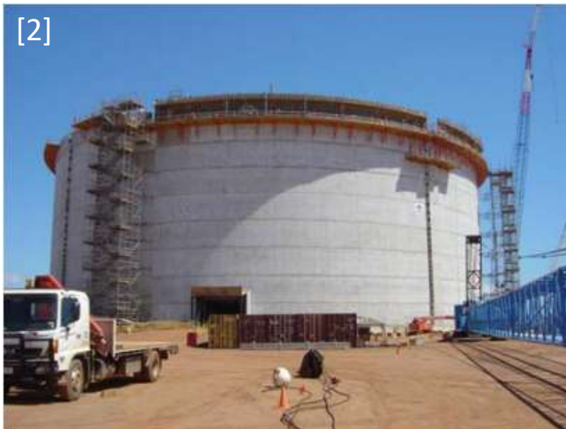
A concrete liquified natural gas (LNG) tank near completion in Darwin, Australia
