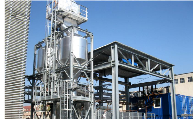
SandTES pilot plant at TU Wien
