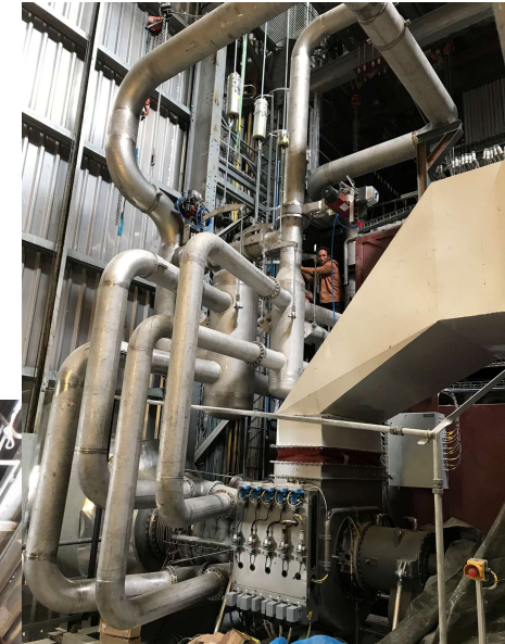
Pressurized air connexion between the heat exchanger and the gas turbine
