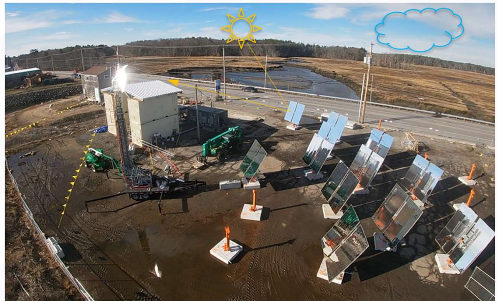
Brayton Energy Solar Test Facility
