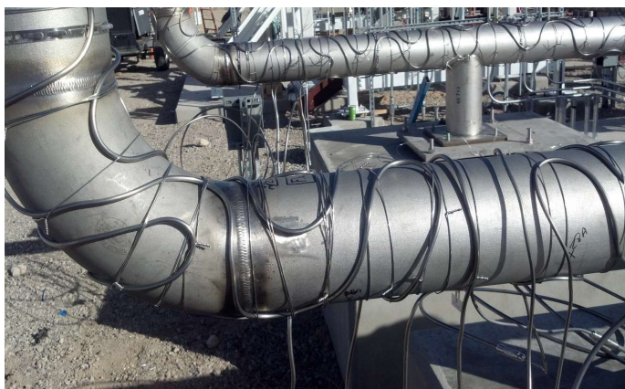
MI cable installation for MSTL at Sandia.
