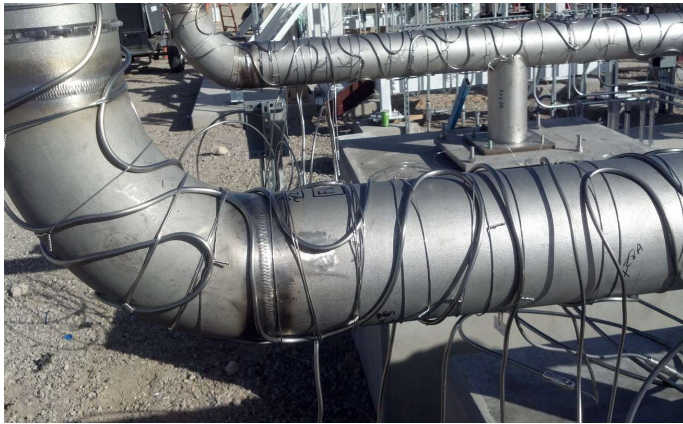
MI cable installation for MSTL at Sandia.
