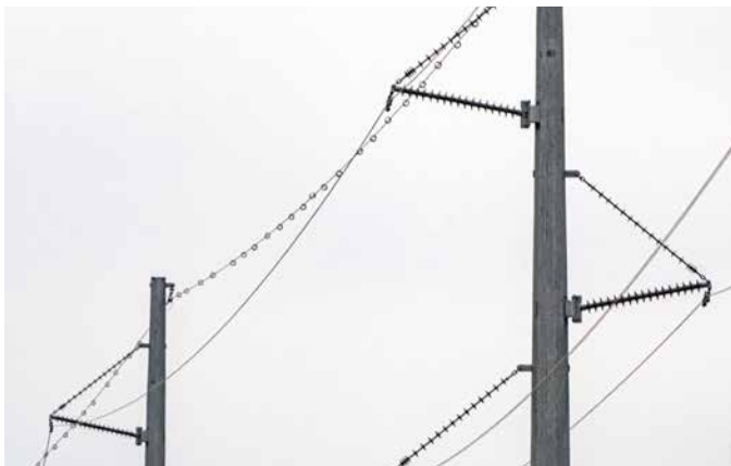
Bird diverters on power poles at the Flatirons Campus substation. The substation is part of the recent Power Generation Upgrade Project. Photo by Werner Slocum, NREL 64460
