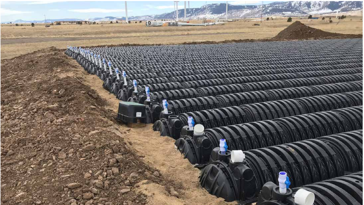
A new onsite wastewater treatment system was installed at the Flatirons Campus in 2020 to replace the original system, which was no longer adequate for the building population it served. The system was permitted through Jefferson County Public Health Department. Photo by Brian Cox, NREL 63269
