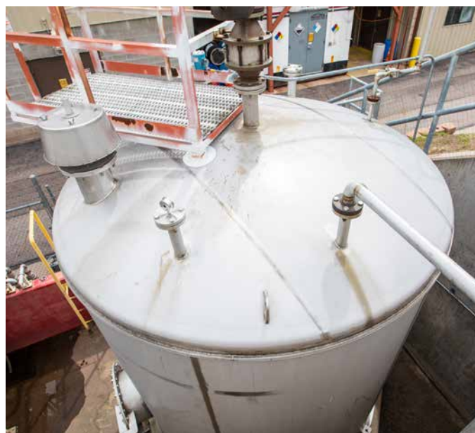
A 6000-gallon (22,712 L) ethanol AST and secondary containment basin on the STM Campus supports research in biomass development. Photo by Werner Slocum, NREL 55981
