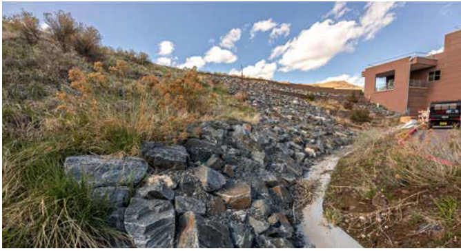
Efforts to stabilize the hillside west of the Field Test Laboratory Building (FTLB) to allow for proper water drainage continues at the STM Campus. Photo by Werner Slocum, NREL 64468
