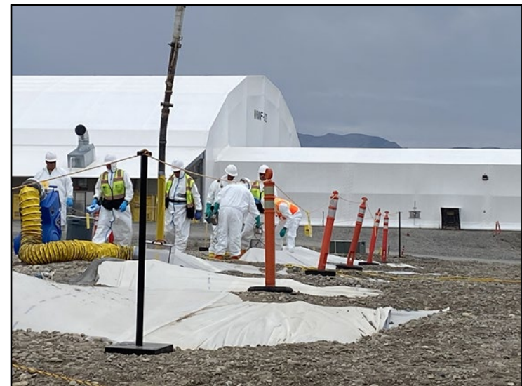
Burial of DPSs – Grouting to fill voids
