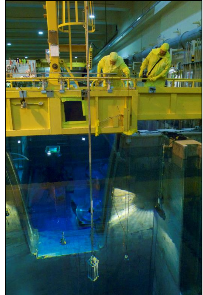
SNF Crew transferring EBR-II fuel to the cask loading pool
