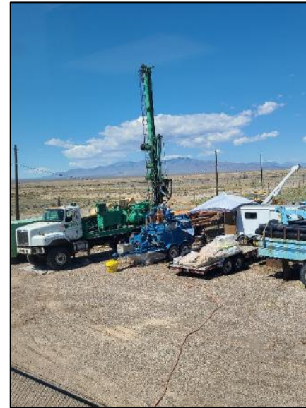
USGS drilling the new ISB treatment well, TAN-2336, and core samples collected from the well
