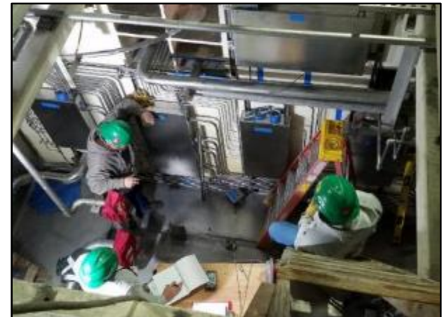
Wet decon control tubing installation inside pipe chase (Pre-COVID)
