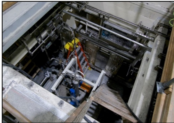
Waste feed pump skid
