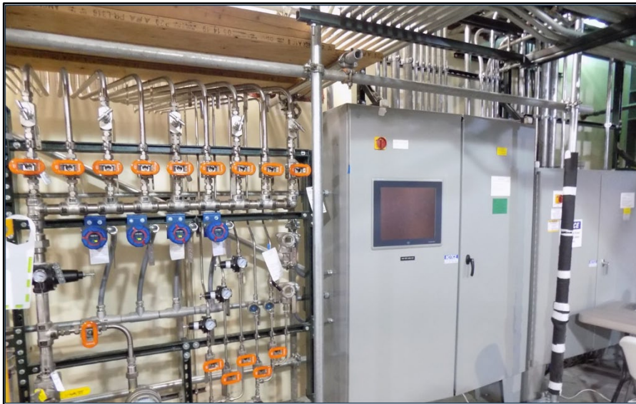
Wet decon system control station
