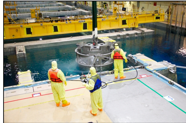
SNF crew removing the fuel-loaded Large Cell Cask from the CPP-666 Basin
