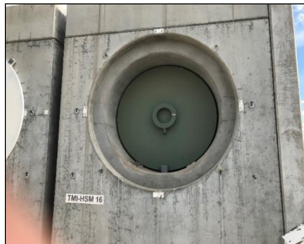
TMI-2 DSC bottom with shielding lid removed
