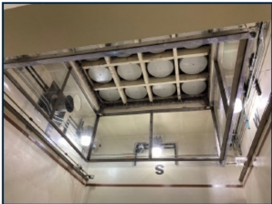
Vault loading cell HVAC plenum
