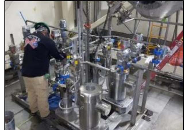
Wet decon system skid installation (Pre-COVID)
