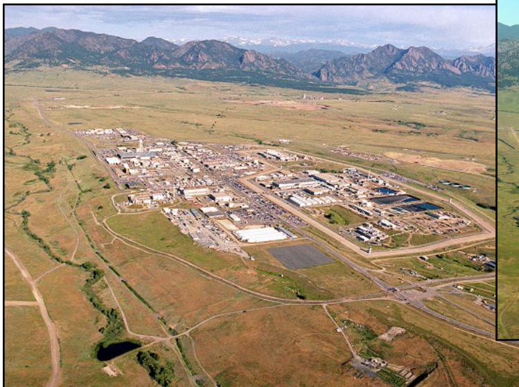
Rocky Flats Site Prior to Final Cleanup (June 1995).
