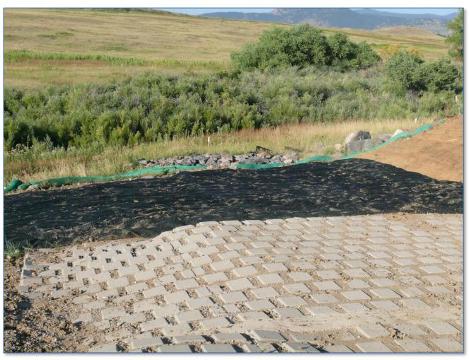
Facing southwest along the East Perimeter Channel, showing erosion control material and articulated concrete blocks. Taken August 14, 2020.
