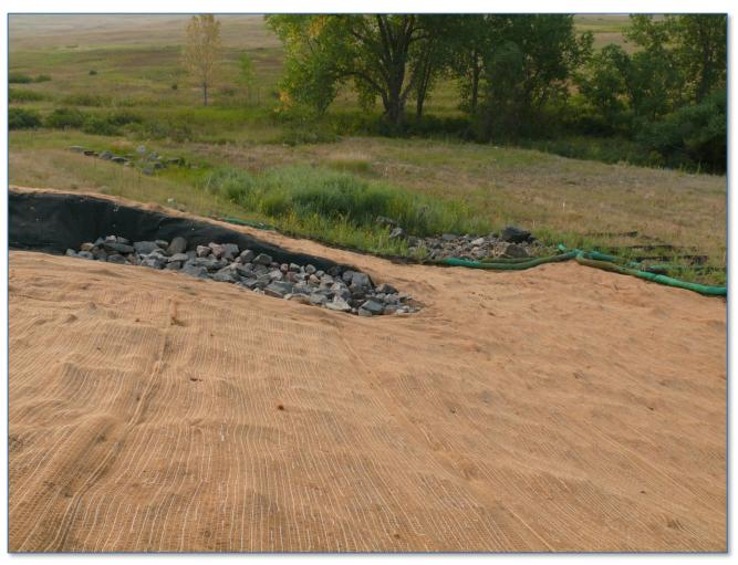
Facing southeast, showing erosion control material. The rock in the foreground is intended to slow water flow. Taken August 21, 2020.
