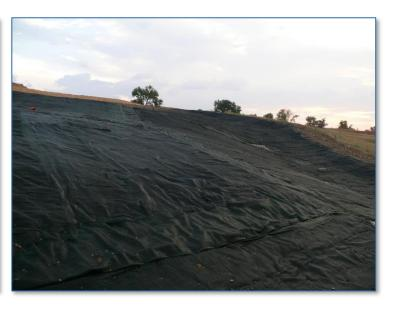
Facing north, showing berms 7 (left) and 6 (center and right), cleanout risers, and erosion control material. Taken Aug. 28, 2020.
