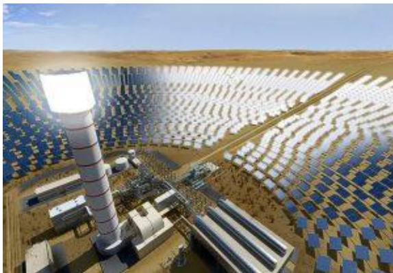
Figure. Silicon carbide fiber composites receiver for high temperature Gen3 CSP plants
