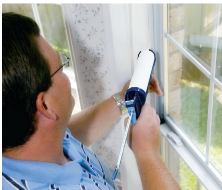
Caulking is one DIY strategy for sealing air leaks.
